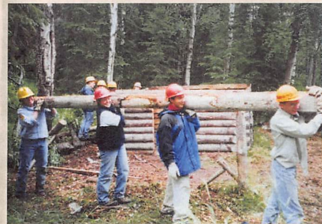
Youth Conservation enrollees dismantling the homestead cabin for boat transport from Tustumena Lake to Soldotna.
