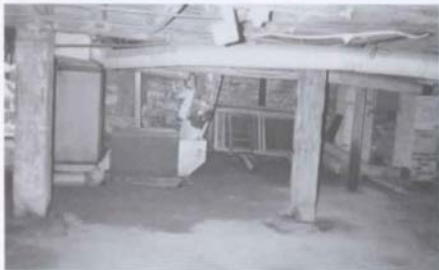
Figure 59. M'Clintock House: Cellar, Interior View Looking Southwest [1988].
