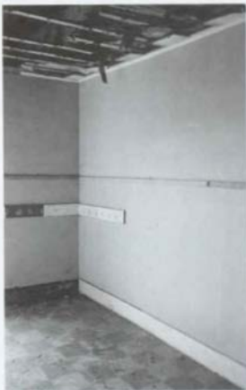
Figure 113. M'Clintock House: Room 204 (Southeast Bedroom), East Half Looking Southwest [1988].
