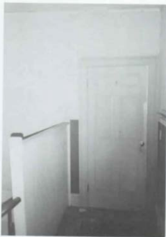
Figure 96. M'Clintock House: Room 201 (Upper Stair Hall), East Side of North Wall, Showing Door Reused from Former Closet [1988].
