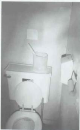
Figure 71. M'Clintock House: Room 101 (Toilet Room Under Stairway), North Wall [1988].
