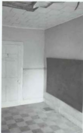
Figure 111. M'Clintock House: Room 204 (Southwest Bedroom), East Half Looking Northeast [1988].
