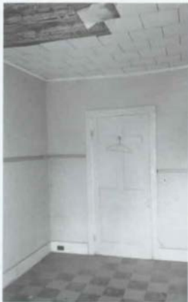
Figure 110. M'Clintock House: Room 204 (Southwest Bedroom), East Half Looking Northwest [1988].
