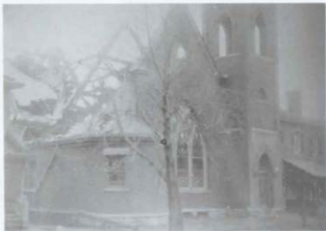
Figure 29. Photograph Showing the Fire-Damaged Baptist Church and Adjacent Parsonage, March 1906.
