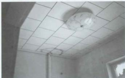
Figure 100. M'Clintock House: Room 201, North End (Toilet Room), Ceiling Looking Northwest [1988].
