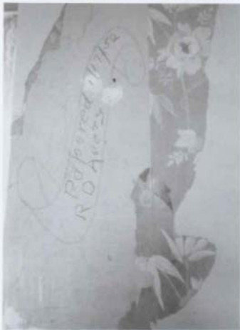
Figure 93. M'Clintock House: Room 104 (Kitchen/Dining Room), Written Note Found Beneath Wallpaper on Chimney Breast [1988].
