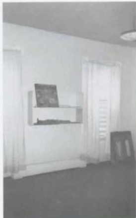
Figure 73. M'Clintock House: Room 102 (Parlor), North Wall [1988].
