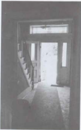
Figure 64. M'Clintock House: Room 101 (Entrance/Stair Hall), Looking North Toward Front Doorway [1988].
