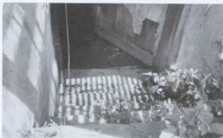
Figure 49. M'Clintock House: South (Rear) Wall, Cellar Steps [1988].
