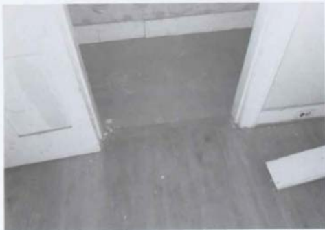
Figure 85. M'Clintock House: Room 103 (Southeast Room), Closet Interior Looking North [1988].
