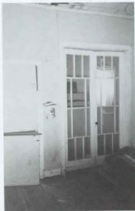
Figure 90. M'Clintock House: Room 104 (Kitchen/Dining Room), North Wall, East End [1988].
