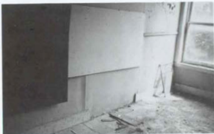
Figure 112. M'Clintock House: Room 204 (Southwest Bedroom), East Half Looking Southeast [1988].
