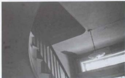
Figure 67. M'Clintock House: Room 101 (Entrance/Stair Hall), Northwest Corner of Ceiling [1988].
