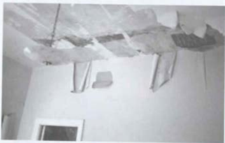
Figure 82. M'Clintock House: Room 103 (Southeast Room), Ceiling at West Wall [1988].
