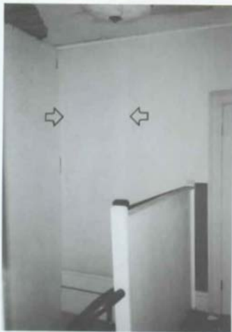
Figure 95. M'Clintock House: Room 201 (Upper Stair Hall), North Wall (arrows show remnant of original closet partition) [1988].
