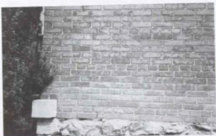
Figure 52. M'Clintock House: West Foundation and Wall, North End [1988].
