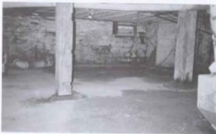
Figure 58. M'Clintock House: Cellar, Interior View Looking Northeast [1988].
