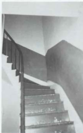
Figure 69. M'Clintock House: Room 101 (Entrance/Stair Hall), Turn of Stairway [1988].
