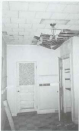
Figure 116. M'Clintock House: Room 204 (Southwest Bedroom), West Half Looking South [1988].
