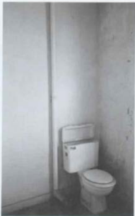
Figure 97. M'Clintock House: Room 201, North End (Toilet Room), Looking Northwest [1988].
