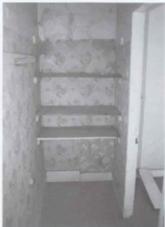
Figure 84. M'Clintock House: Room 103 (Southeast Room, Closet Interior Looking East [1988].
