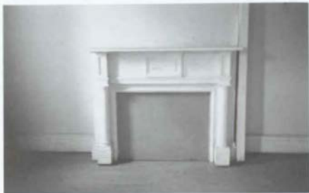
Figure 76. M'Clintock House: Room 102 (Parlor), East Wall, Chimney Breast and Fireplace Mantel [1988].
