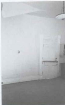
Figure 72. M'Clintock House: Room 102 (Parlor), West Wall [1988].
