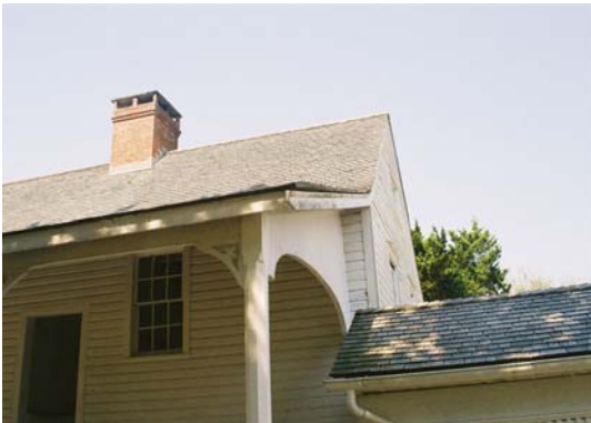
Figure 13: Connection between Breezeway and Kitchen House. (Photo by author.)
