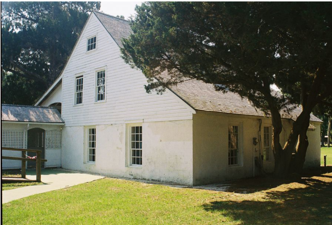
Figure 8: Kitchen House, looking southeast. (Photo by author.)
