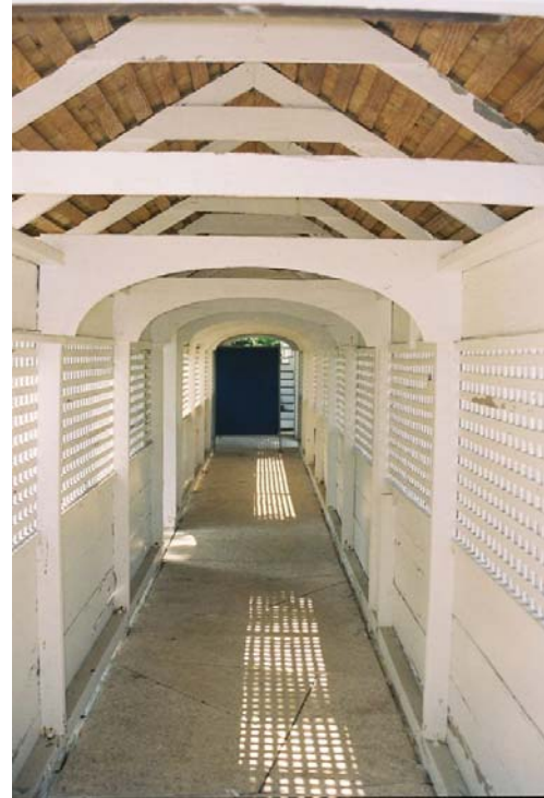
Figure 11: Interior of Breezeway, looking south. (Photo by author.)
