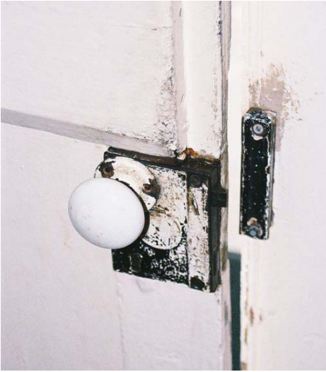
Figure 38: Door 1, white porcelain knob and iron rim lock. Note that the lock is stamped "A&D Manufacturing, Co. May 29, 1866." (Photo by author.)
