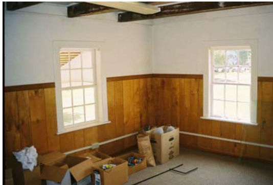
Figure 76: Room 203, looking southeast. (Photo by author.)
