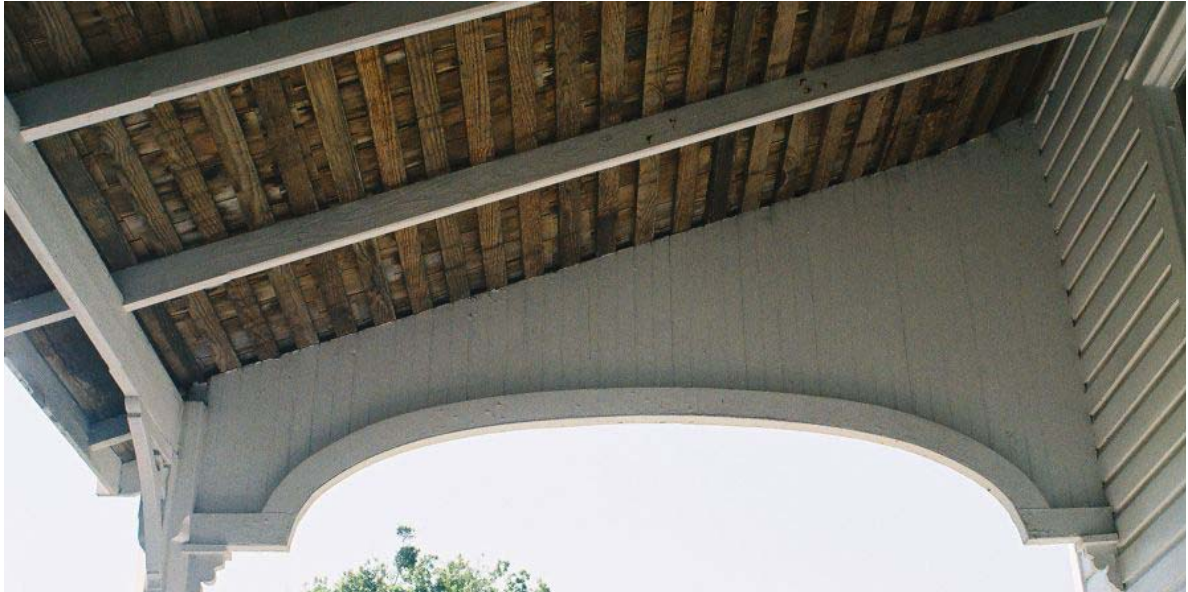
Figure 30: Detail of vertical siding on end of porch roof and drop siding on exterior walls. (Photo by author.)
