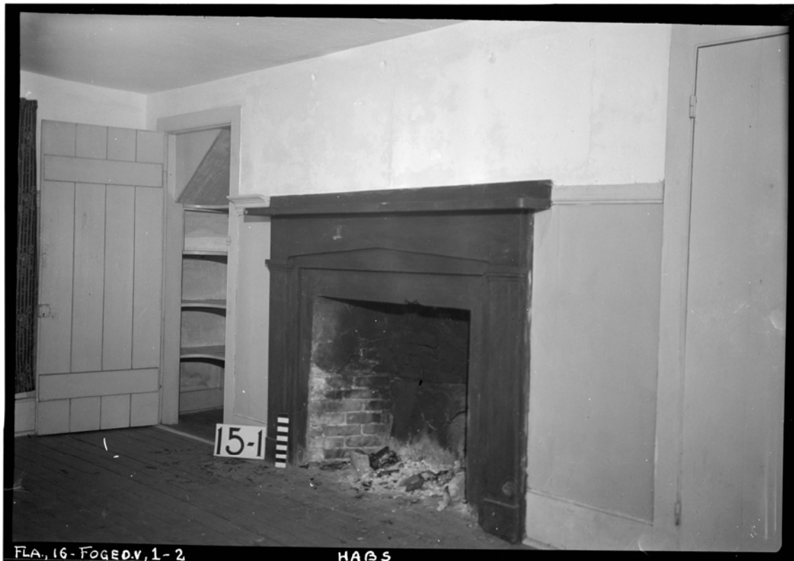
Figure 2: 1934 HABS photograph of Room 101. Note the closets, finished ceiling and molding on either side of fireplace. (Library of Congress.)
