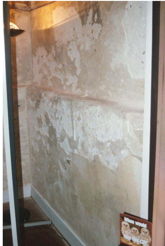
Figure 67: South wall of Room 104. Note ledge which wraps around to east wall. (Photo by author.)
