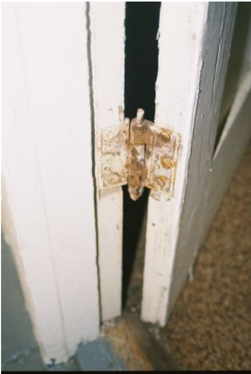
Figure 48: Butt Hinge, Type 5. (Photo by author.)
