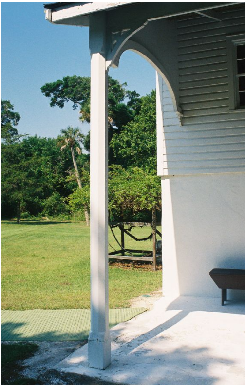
Figure 58: Chamfered porch post. (Photo by author.)
