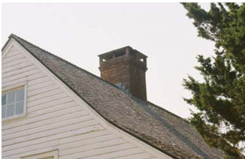
Figure 29: View of shingle roof, drop siding and chimney. (Photo by author.)
