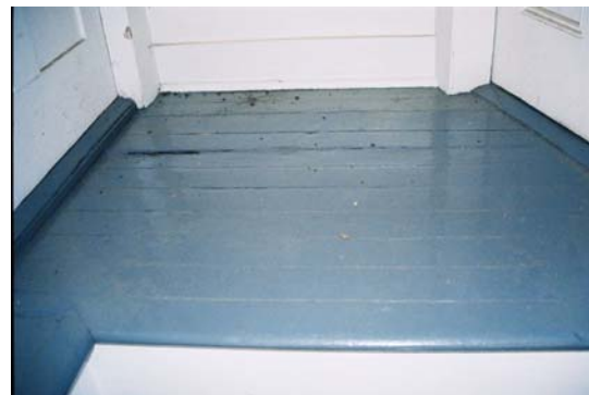
Figure 72: Landing at top of staircase. (Photo by author.)
