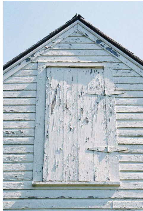
Figure 37: Door 16, a modern board-and-batten door. (Photo by author.)
