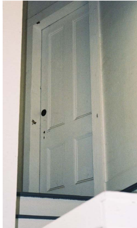
Figure 35: Door 11, a four-panel door. (Photo by author.)
