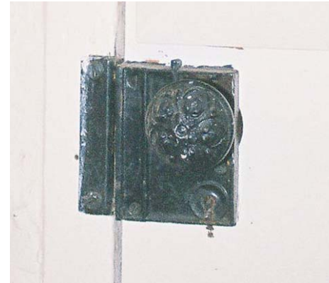
Figure 43: Door 8, interior embossed metal knob and rim lock. (Photo by author.)
