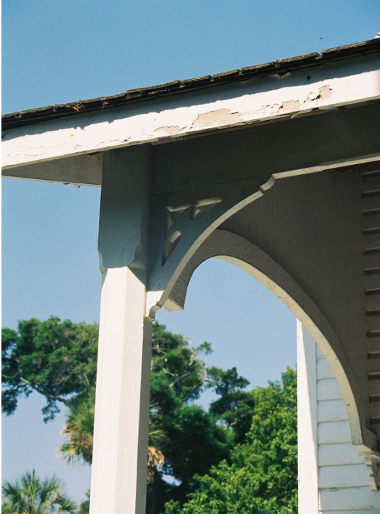
Figure 60: Detail of porch roof bracket. (Photo by author.)
