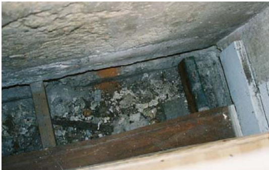
Figure 16: Exposed floor joists above sand/shell grade in Room 104. (Photo by author.)
