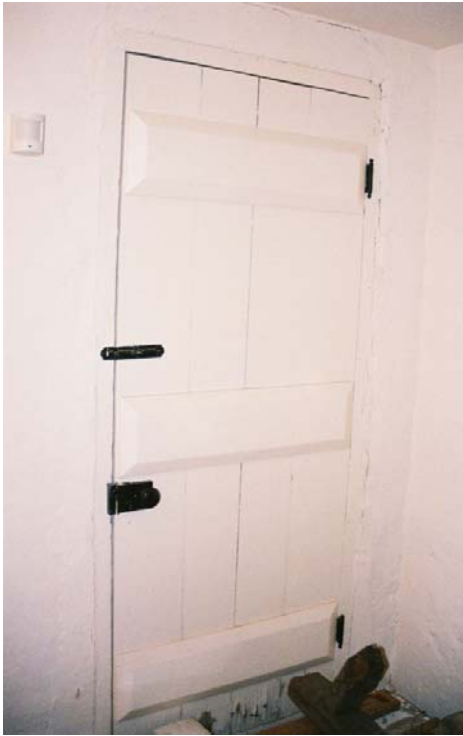
Figure 34: Door 7, a typical board-and-batten door. (Photo by author.)
