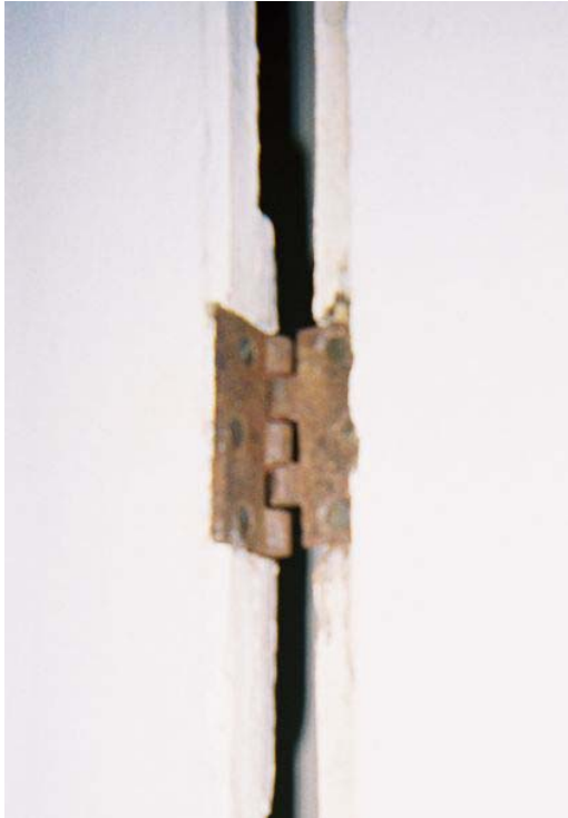
Figure 44: Butt Hinge, Type 1. (Photo by author.)
