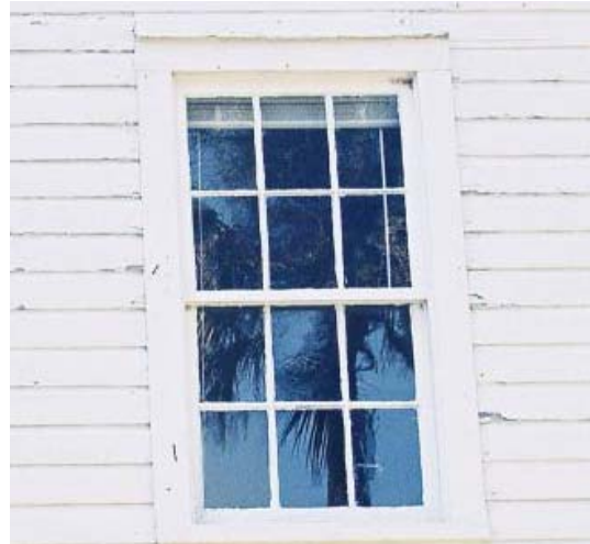
Figure 54: Window 14, example of 6/6 window, typical to the second floor. (Photo by author.)
