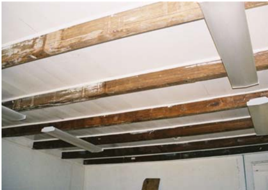
Figure 23: Floor joists of attic space above Room 203. (Photo by author.)
