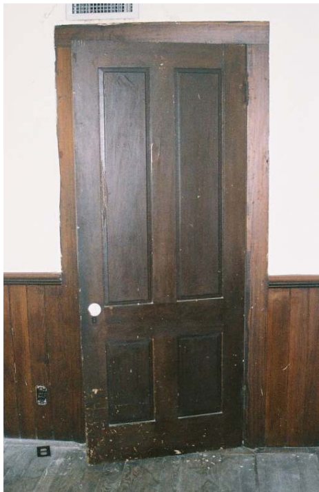
Figure 36: Door 12, a four-panel door. Note the raised panels. (Photo by author.)
