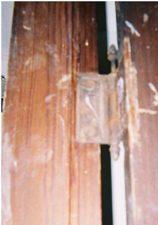
Figure 46: Butt Hinge, Type 3. (Photo by author.)
