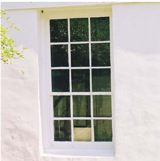
Figure 53: Window 7, example of 9/6 window, typical to first floor. (Photo by author.)
