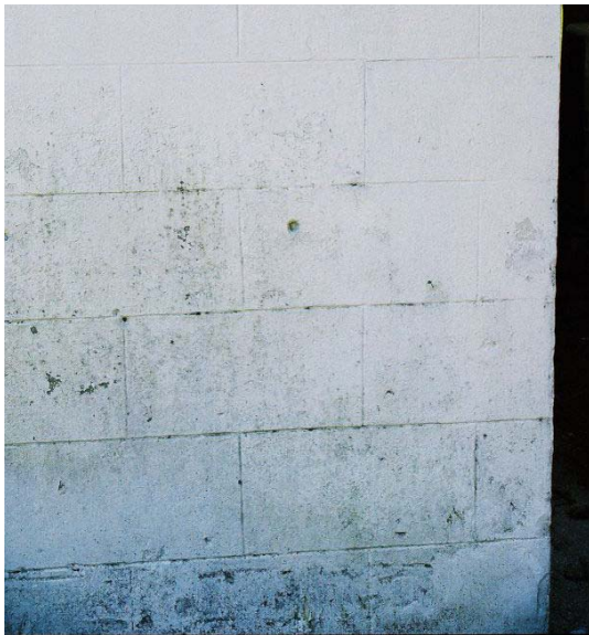
Figure 31: Detail of stucco wall, scored to resemble ashlar masonry joints. (Photo by author.)
