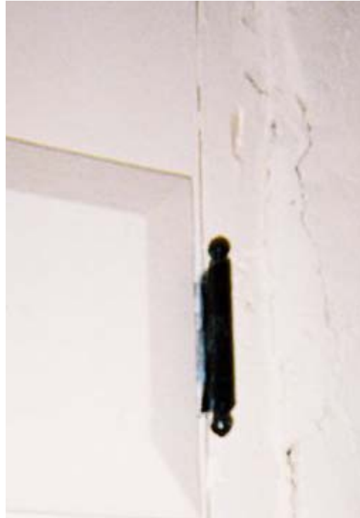
Figure 45: Butt Hinge, Type 2. (Photo by author.)
