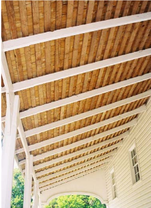
Figure 28: Porch rafters. Note that the shingle lath and shingles have been replaced. (Photo by author.)
