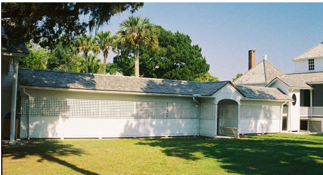
Figure 12: Breezeway between Main House and Kitchen House. (Photo by author.)
