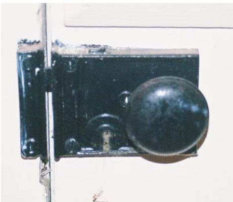
Figure 42: Door 7, interior metal knob and rim lock. (Photo by author.)
