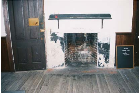
Figure 73: Room 201, looking south. (Photo by author.)
