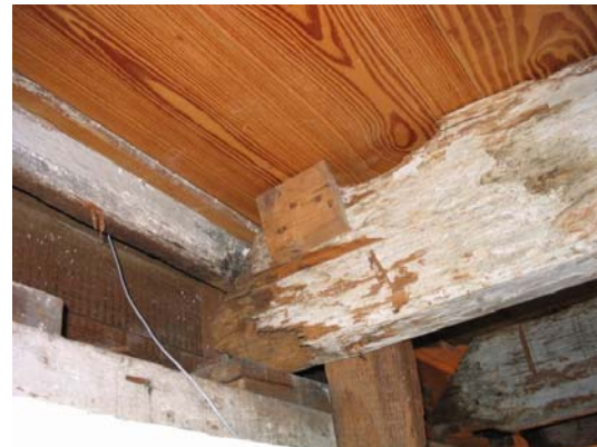
Figure 22: Hewn joist bearing on supplemental sash sawn beam and masonry wall. (Photo by author.)
