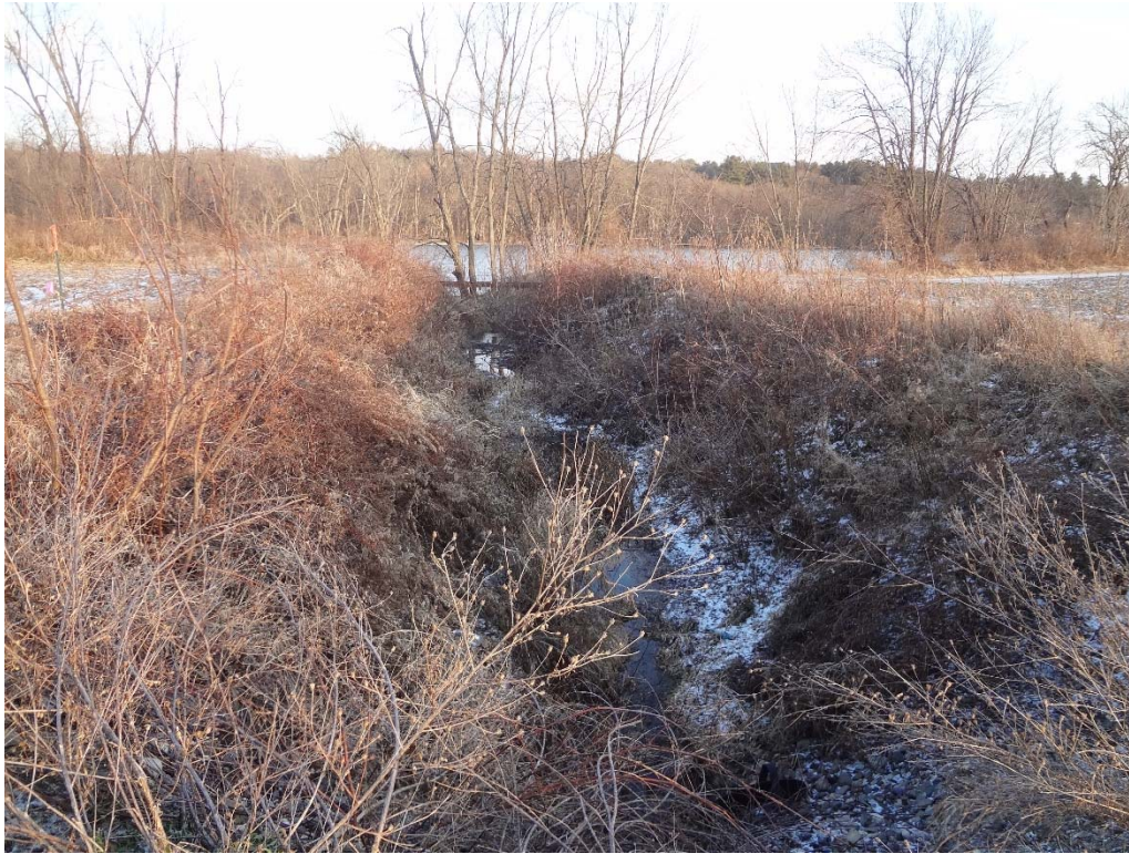
Photo 3. A man-made east-west aligned drainage near its confluence with the Hudson River (visible in the background). The drainage may have followed a natural system, but has been straightened and deepened over the years to protect this valuable farm land from flooding,
