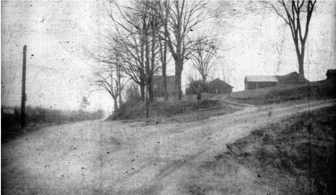
Figure 14. View looking south at Chubbs Hill Road (Schuyler Street) and Whitehall Turnpike (US Route 4), ca. 1920s. Allen House (Hartloff House) and agricultural outbuildings in the background. A person stands near the surrender marker. To their right is one of the driveways to the Germain property, possibly the trace of the old Road to Albany. (Saratoga NHP Archives; from CLI draft 2008: 162)
