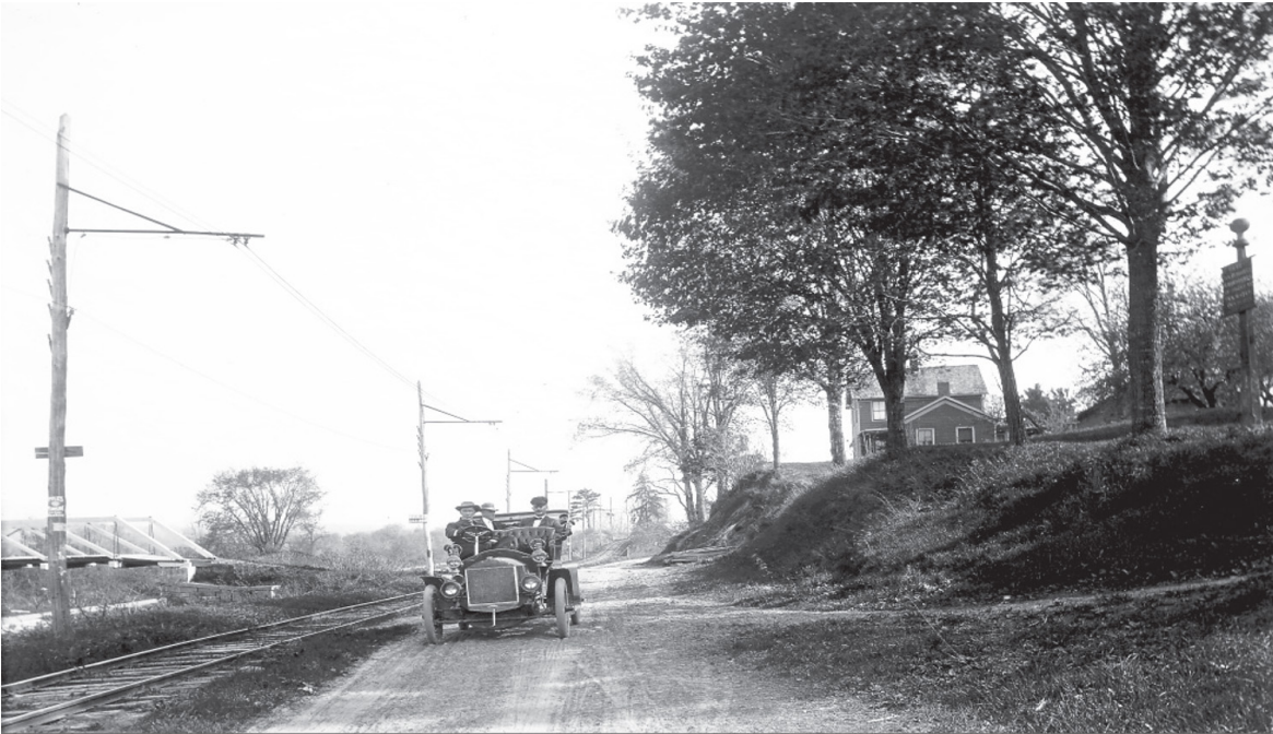
Figure 11. View looking south along the Whitehall Turnpike, ca. 1910-1915. At image right are the Saratoga Historic Surrender Marker, intersection of Schuyler Street and Whitehall Turnpike (U.S. Route 4), and Cora B. Allen House. To image left is Bridge No. 58, the Champlain Canal, and Hudson Valley Electric Railroad. ( Saratoga NHP Archives, from CLI draft 2008: 55 )
