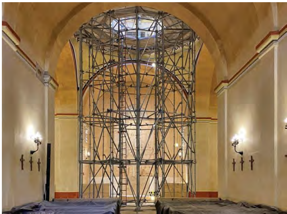
Restoration work at Mission Concepción
