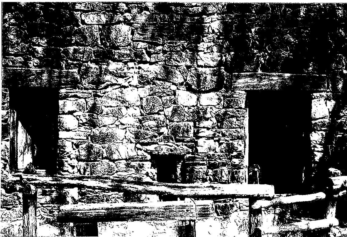
Figure 2-64 March 1979. View of the south elevation of the mill. Note the upper portion of the sluice gate frame still intact. Courtesy of the Texas Parks and Wildlife Department.
