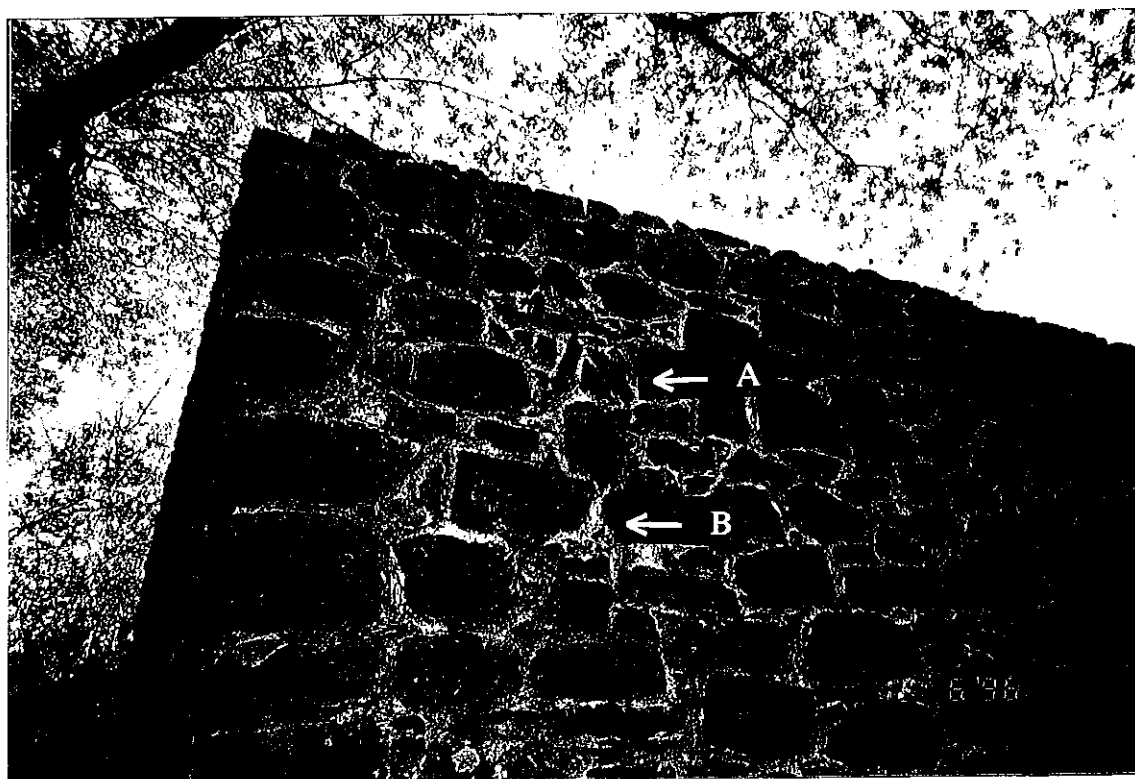
Figure 3-29 December 6, 1996. Detail of upper northeast elevation indicating possible presence of removed wooden drain in this location. Arrow "A" points to inverted "V" arrangement of flagstones used in the 1930s to form a lintel-arrangement above all wooden drains installed at that time (see Figure 3-34). In the 1960s, during the re-roofing of the mill and Indian quarters at Mission San José, all wooden drains were closed off (the mill's were also removed) and concrete drains formed to resemble wood, were installed. Arrow "B" points to tar drips immediately below this inverted "V" indicating that a drain did indeed exist at this location.
