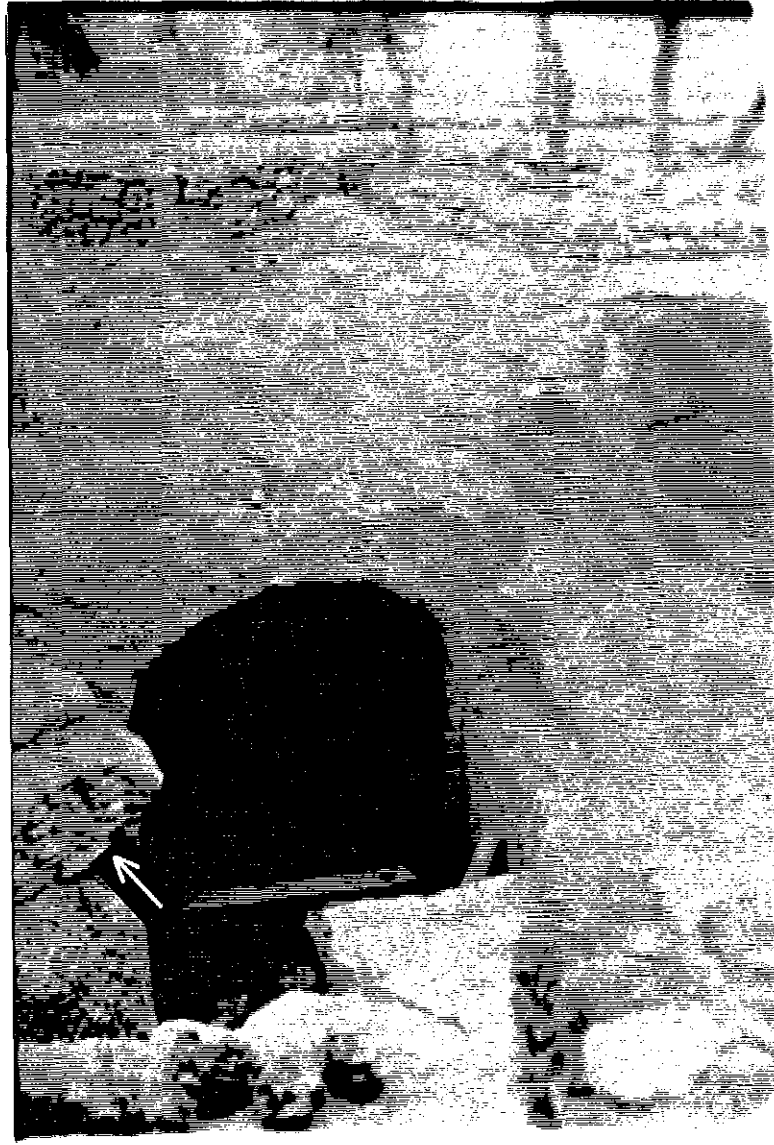
Figure 2-22 ca. 1934. Looking south toward the turbine room opening. A few stones from the mill race (presumably historic) can be seen at the lower left (arrow). The "tail" of the arrow appears to point to a wooden element approximately the shape of a bridge tree, however, this has not been documented.
