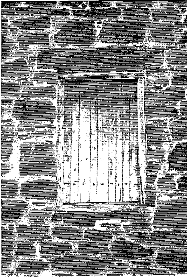
Figure 3-48 June 1996. Detail of the window/shutter in the north elevation.
