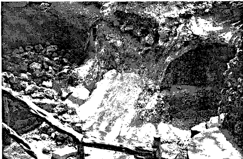
Figure 2-70 ca. 1982. View of the north exterior elevation. The change in masonry immediately below the concrete canal in the upper center of the photograph is very obvious in this photograph supporting the change from three drains to a single one in the 1950s (refer to Figure 3-35).
