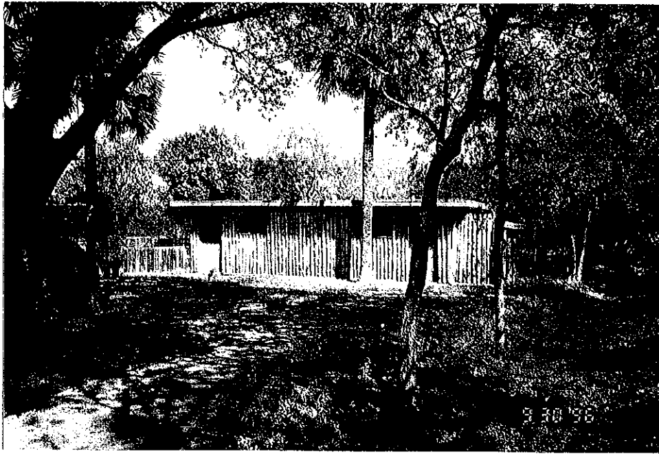
Figure 3-22 September 1996. Modern (ca. 1970) concrete block dressing room which has been sheathed in halved cedar logs in an attempt to help blend the structure with its surroundings. This structure sits almost due east of the mill and is a modern intrusion into the historic scene. The acequia, which terminates just south of the building, can be seen in the lower right corner of the photograph.
