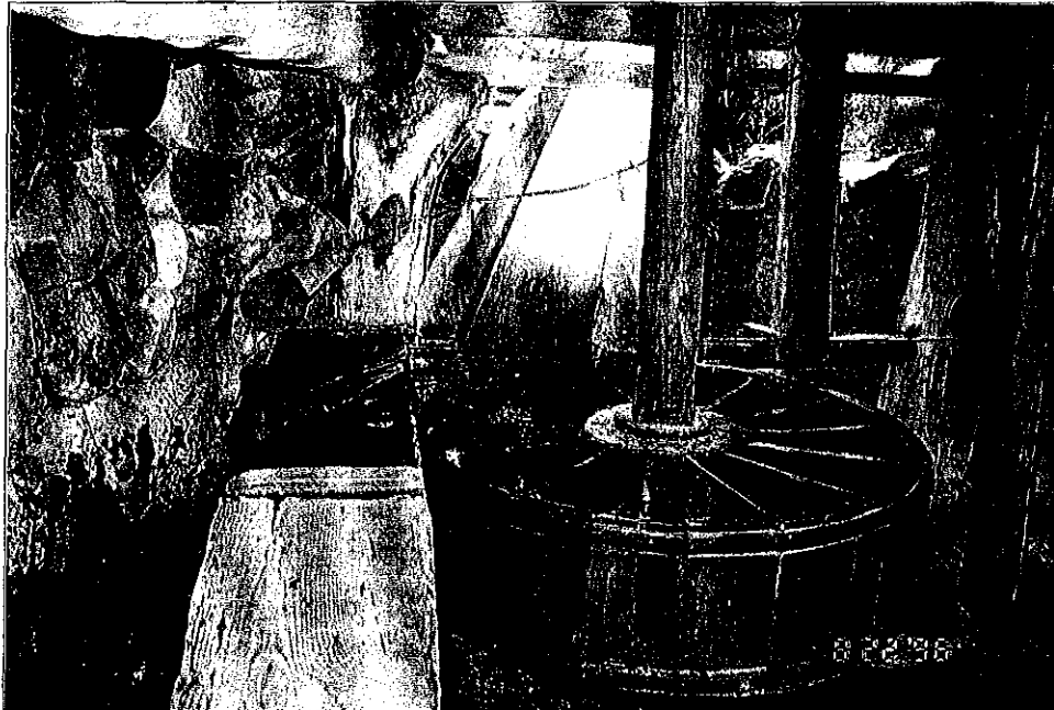
Figure 1-41 August 22, 1996. Water has been introduced into the acequia and wooden aqueduct for a demonstration. Here it is being diverted via the diverter board, away from the wheel (the "on-off" water control for the restored Truchas mill). One of the two pulleys which control the diverter board can also be seen at the left center of the photograph. El Rancho de las Golondrinas, Santa Fe, New Mexico.
