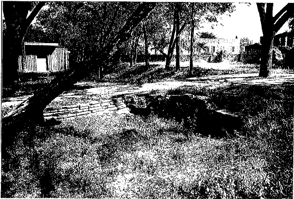
Figure 3-11 September 30, 1996. View of masonry retaining wall (non historic) which acts like a weir directing acequia madre water through a culvert under a modern brick walk south of the mill. The modern dressing room pictured in Figure 3-22 can be seen at the upper left of the photograph.
