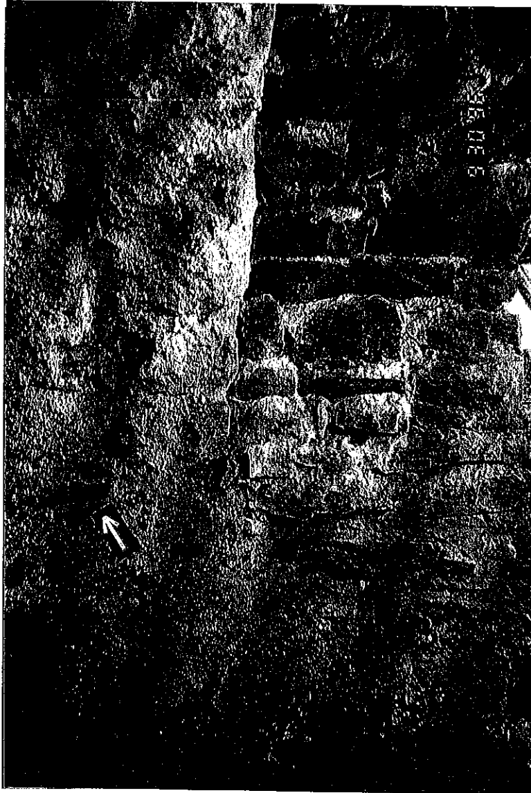
Figure 3-67 September 25, 1996. Looking northwest along the junction of the historic wall/parging (at the left of the photograph) and the 1930s restoration masonry. The arrow points to another gate hinge pin.
