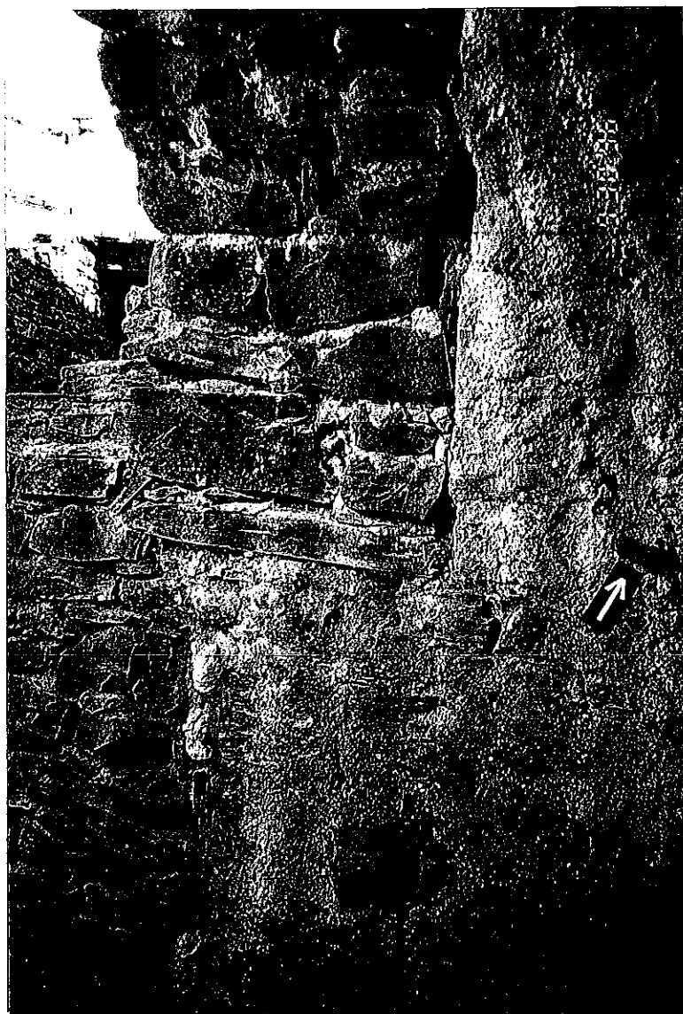
Figure 3-66 September 30, 1996. Looking southeast along the junction of the historic wall/parging (at the right of the photograph) and the 1930s restoration masonry. The joint between old and new is obvious. The arrow points to what looks to have been a hinge pin for a metal gate which shows up in one of the historical photographs associated with the San Antonio Express newspaper article, July 23, 1937 (Figure 2-45). There are four pieces of metal sticking out of the wall, two on either side that would have held the gate.
