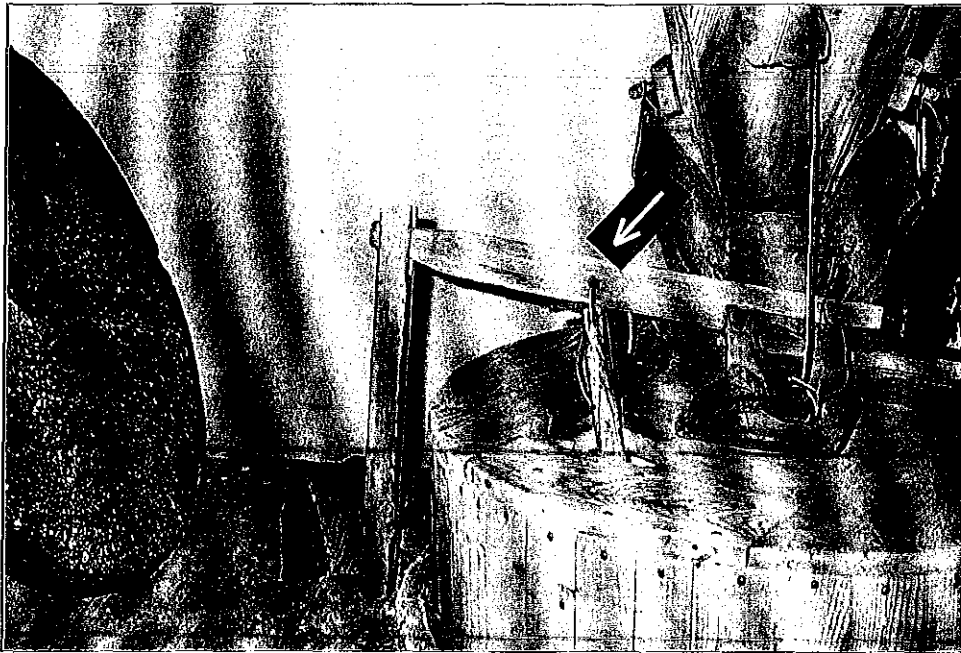
Figure 1-71 August 22, 1996. The "dancing damsel" (see arrow), which is inserted through the casing, rests on the table and is connected to the hopper/chute assembly and acts as a vibrating mechanism to keep the unground grist moving down the wooden chute from the hopper into the denim chute below. The small wooden dowel which is inserted through the casing sits atop the rotating top stone and as the stone rotates, it bounces along the rough surface, carrying that vibration to the wooden chute below the hopper.
