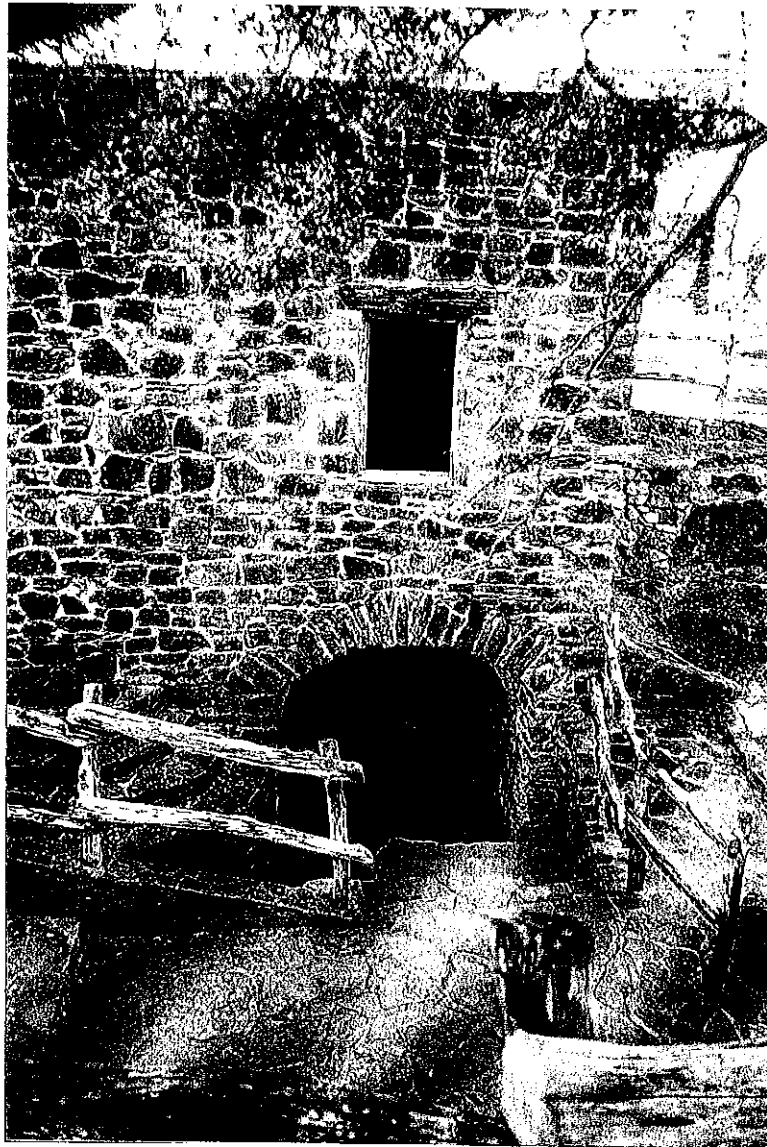
Figure 3-47 June 1996. Overall north elevation of the mill. There is one shuttered window at the northwest corner. The arched stonework above the wheel room vault can be seen at the lower right of the photograph.
