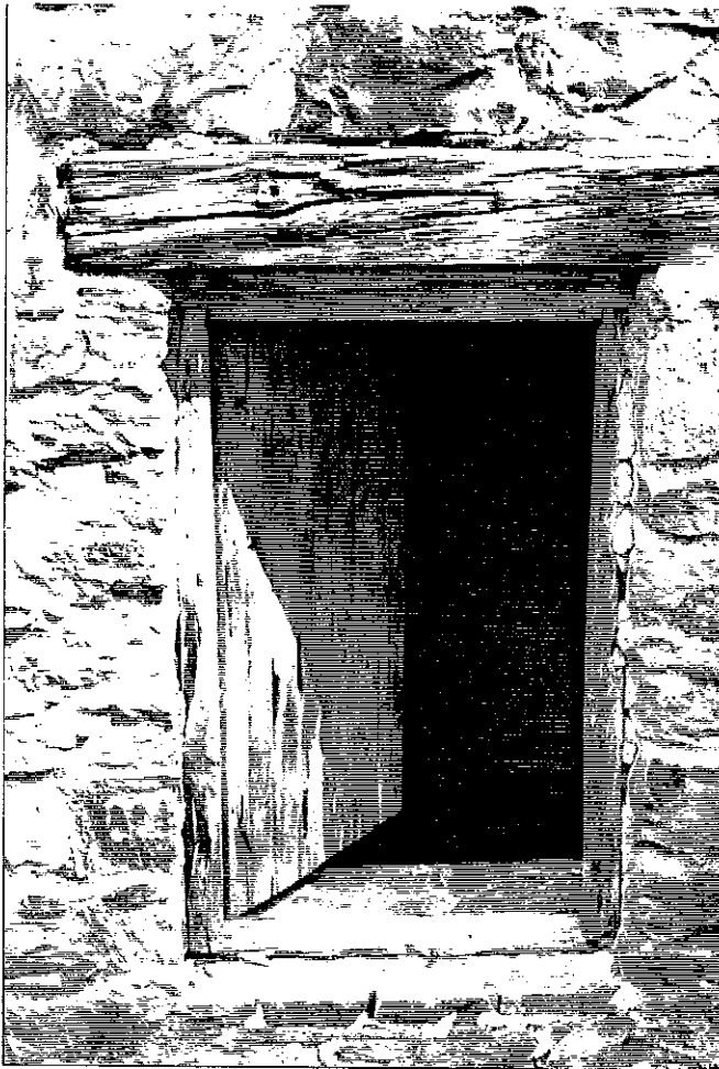
Figure 3-39 June 1996. Detail of the middle window in the south elevation. The condition of the lintel is fair to good, minor pointing is required, primarily above the window lintel.
