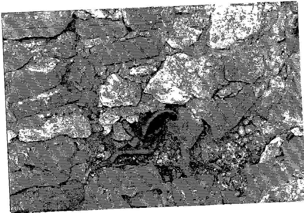
Figure 3-143 June 1996. Detail of a clay drainage tile, which comes from "tanning" vat to the south. Note: It looks like a section of the masonry millrace was taken out to put in the terra cotta drainage pipe.
