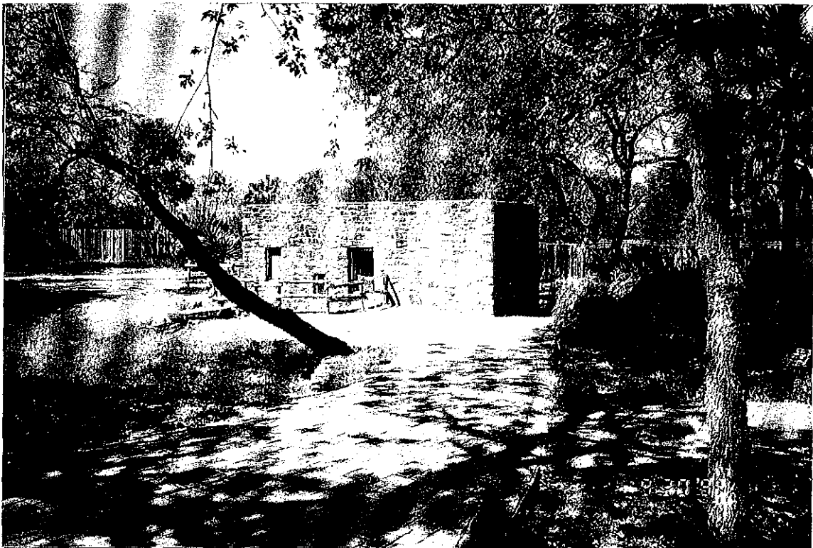
Figure 4-1 September 30, 1996. South elevation of the mill showing the modern brick walk which approaches the mill from the south part of the Mission San José complex.
