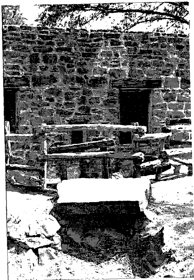
Figure 2-67 1981. Close-up view of the south elevation. Note the flagstone crossing and sluice gate frame. Compare this photograph to Figure 3-36.
