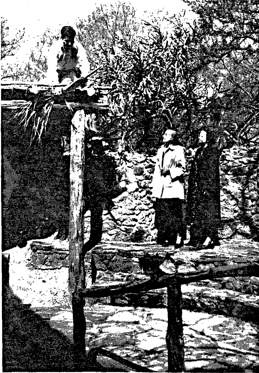
Figure 2-56 April 16, 1950. "Angel Rendon shows Mrs. Hubert Pouquet, Mrs. E.C. Wood how to thatch." (From the San Antonio Express Magazine ). This is a second photograph located which helps provide details for the missing shed roof over the lime kilns. Courtesy of the Daughters of the Republic of Texas Library.
