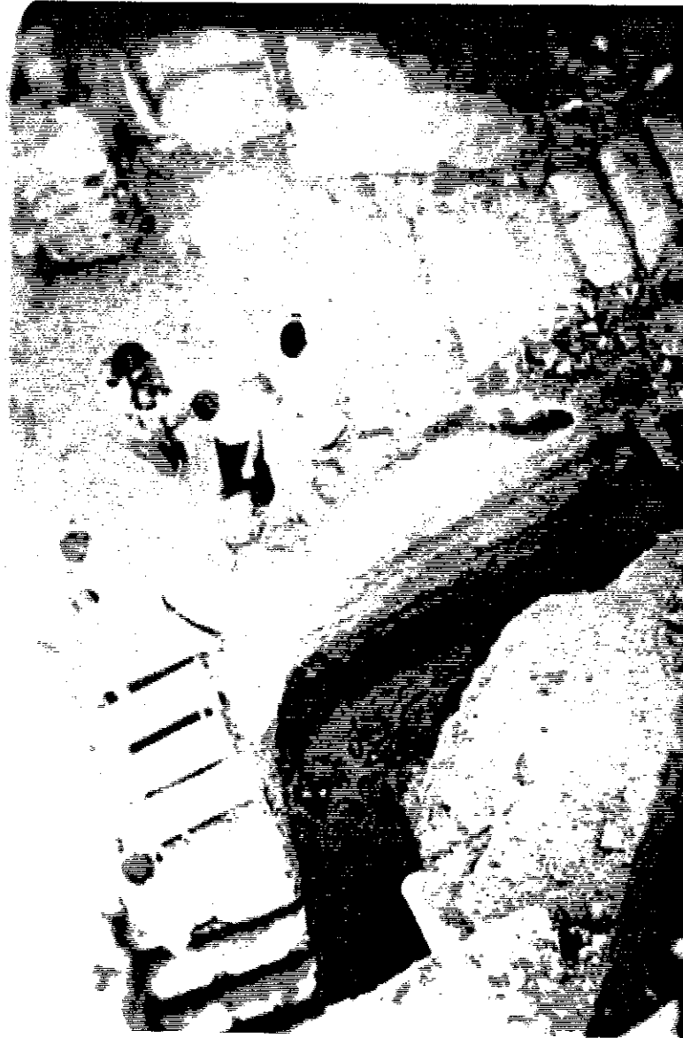
Figure 2-24 ca. 1934. Looking down into the mill race, which has been totally excavated. The stone steps out of this lower area can be seen at the upper right, and the steps down into the wheel room at the lower left. Temporary wooden steps have been installed immediately above the stone steps.
