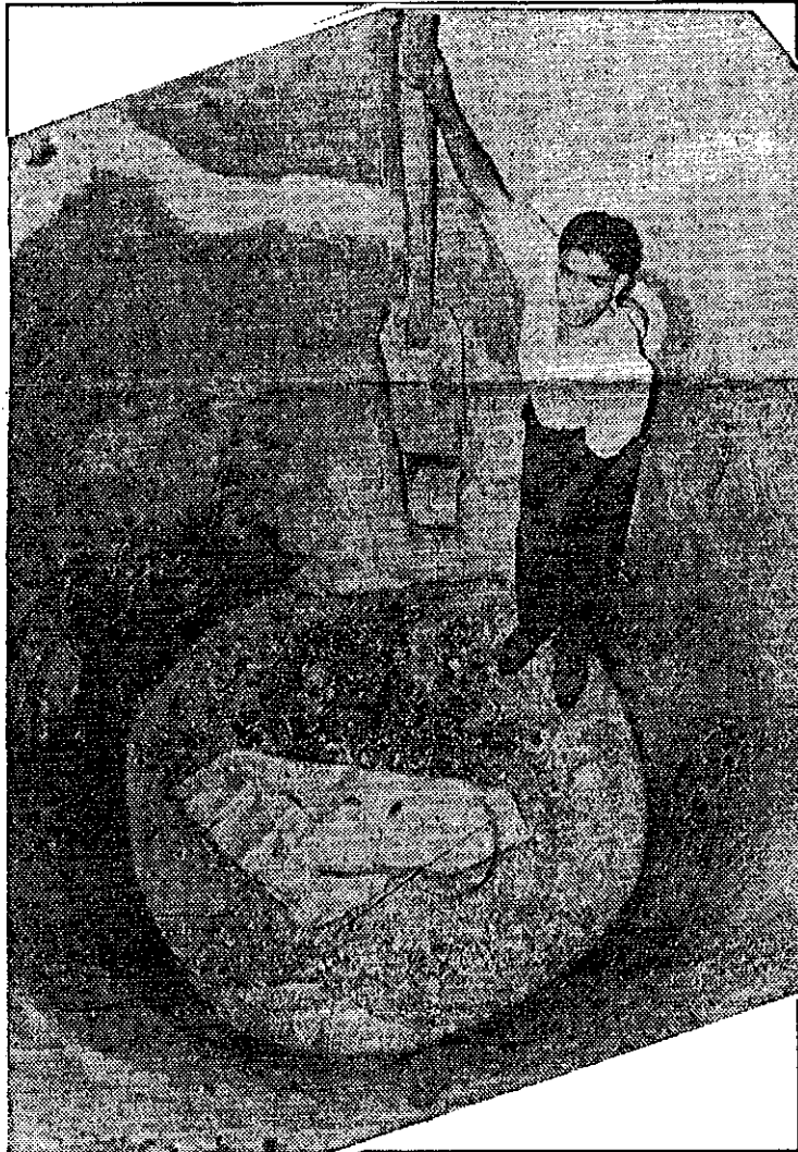
Figure 2-48 March 18, 1938. Photo from the San Antonio Light of the newly restored mill, looking into the forebay. The caption read, "B. Vallejo in sluice pit raises sluice gate letting water into bottom of mill through wooden pipe." (If this was true, Mr. Vallejo would be standing in water). This photo does give a good view of some of the operating mechanism particularly the forebay gate and attached control arm. Courtesy of the Daughters of the Republic of Texas Library. (The photo was cropped in the newspaper article).
