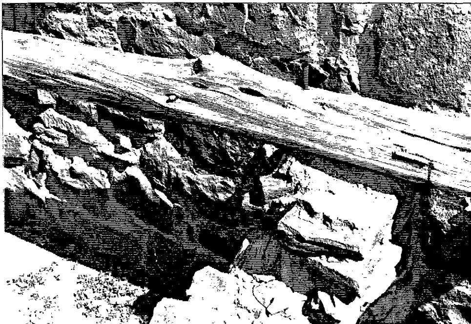
Figure 3-133 June 1996. Looking south along the west elevation. Remnants of the shed roof which was installed over the lime kilns in the 1950s (for protection). A wooden beam with ferrous bolts attached to it rests across viga-like wooden posts coming out of the west elevation of the building. At the back of the photo, just below the rails of the cedar fence, is a short masonry wall which slopes to the west and comes to rest at another very short masonry wall with another wooden beam still embedded in it (see Figures 3-137 and 3-138).
