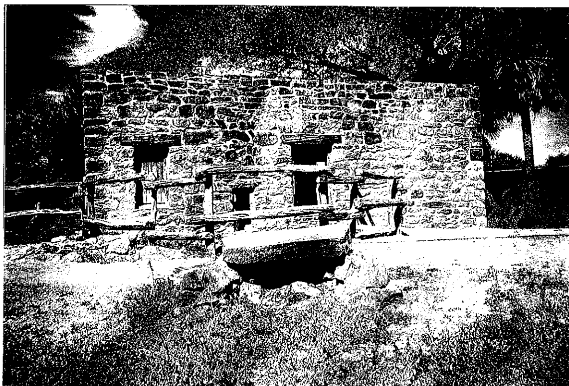
Figure 3-36 September 30, 1996. Overall south elevation. Note the huge slab of sandstone spanning the sluice. This stone (or one similar) is indicated in Smith's 1937 site plan of the mill area (Figure 3-4).
