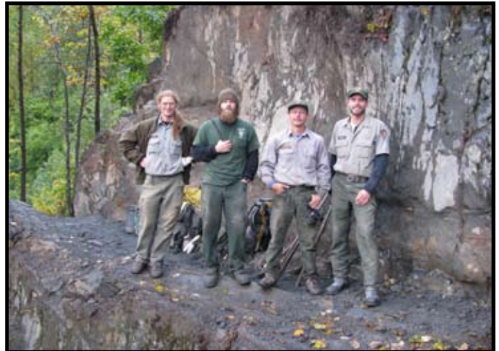
Jeremy Long, Tim George, Dave Larsen, and Luke Henry work on the Harding Icefield Trail in Kenai Fjords National Park.
