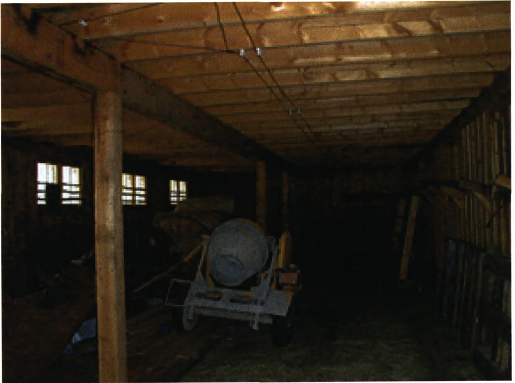
East room – existing conditions
