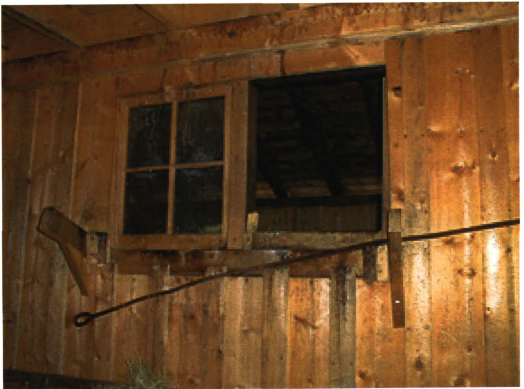
Interior wall – East room – existing conditions
