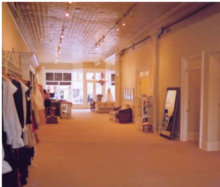
Retaining historic character: The historic tin ceiling was retained during the rehabilitation for this Main Street clothing store.
