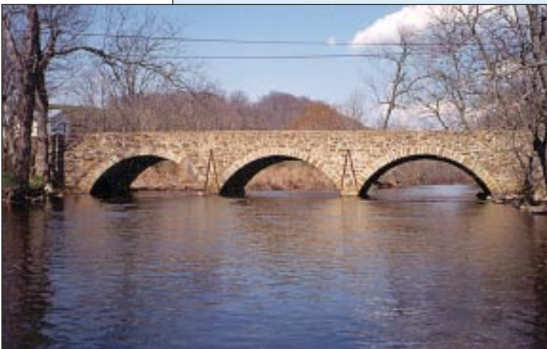
Old Turnpike Road Bridge
