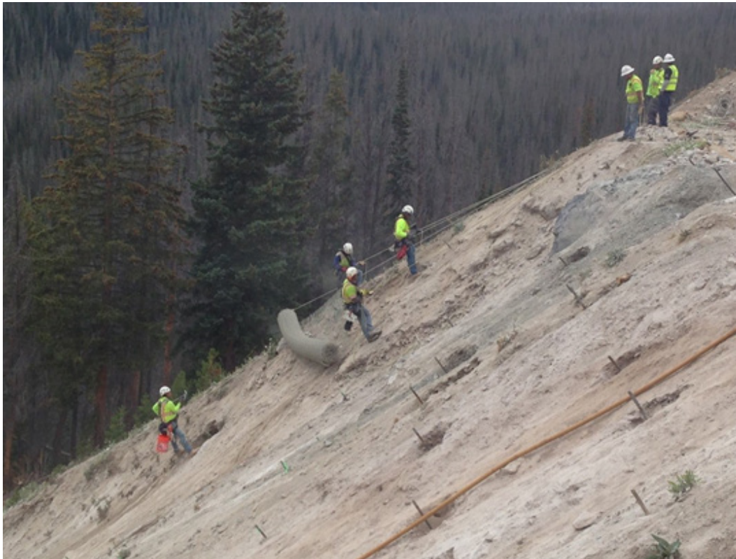
Figure 1. Workers stabilize a hillside in Rocky Mountain National Park below the Grand Ditch.
