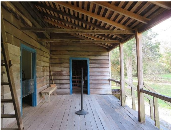
Photo 44. North gallery, looking west.
