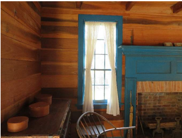
Photo 248. Window W200 from the interior.
