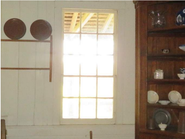
Photo 241. Window W100 from the interior.
