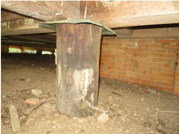
Photo 173. Pier P12, looking northwest.
