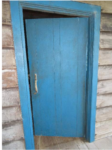
Photo 140. Door D300, overall with door partially closed.
