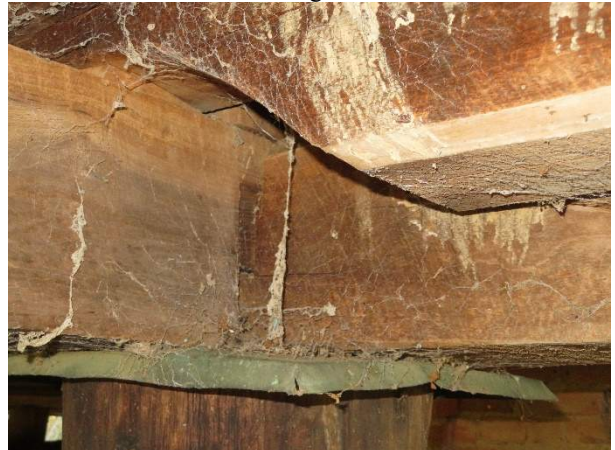
Photo 174. Detail of copper flashing cap at Pier P12.
