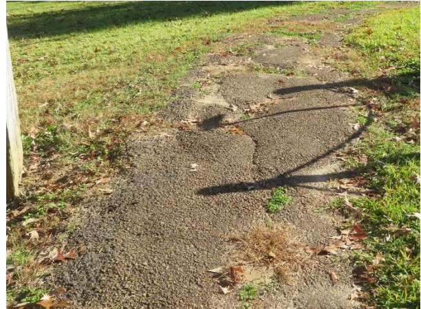
Photo 7. Paved walkway on north side of house, showing cracked and uneven paving.
