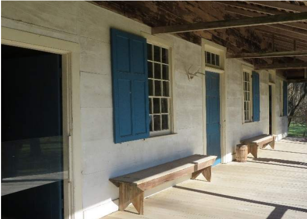
Photo 55. South elevation board siding.
