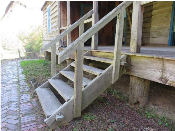
Photo 35. Exterior stairs to north gallery.
