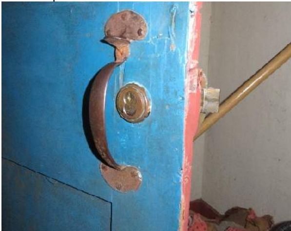
Photo 147. Exterior door hardware.
