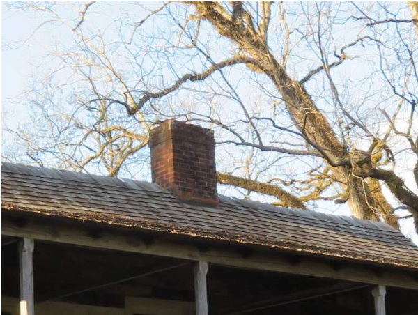
Photo 73. Central chimney above roof, south face.
