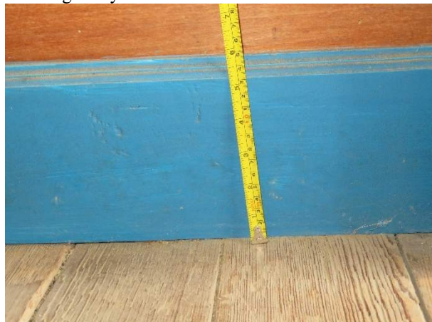
Photo 311. Simple base board.
