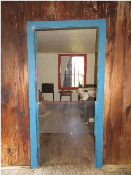
Photo 145. Door D600 with plexiglass pedestrian barrier in place.
