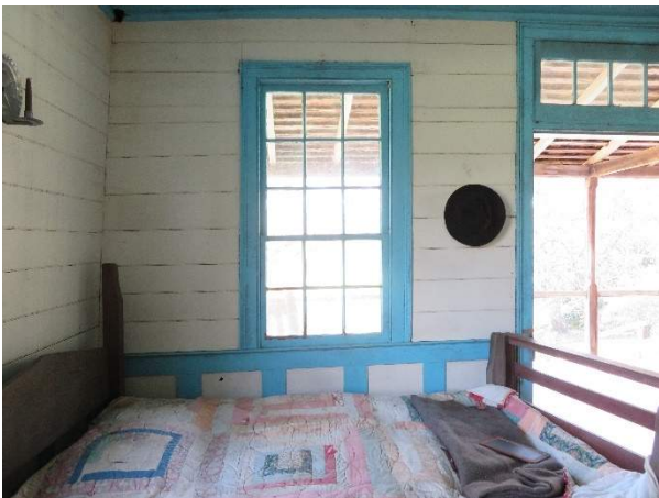
Photo 261. Window W700 from the interior.
