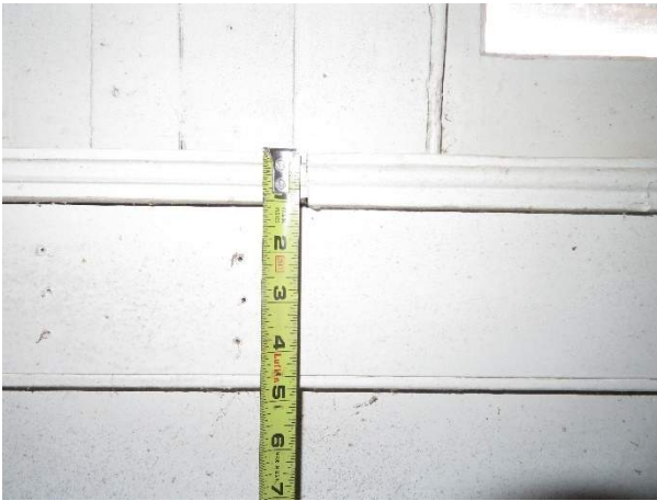
Photo 302. Chair rail moulding profile on the south wall.
