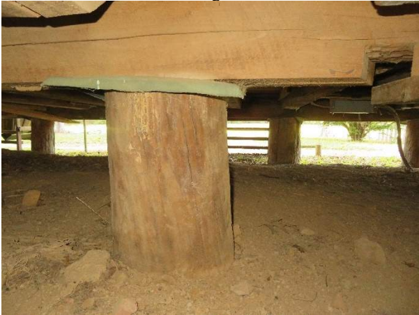
Photo 181. Pier P18, looking north.
