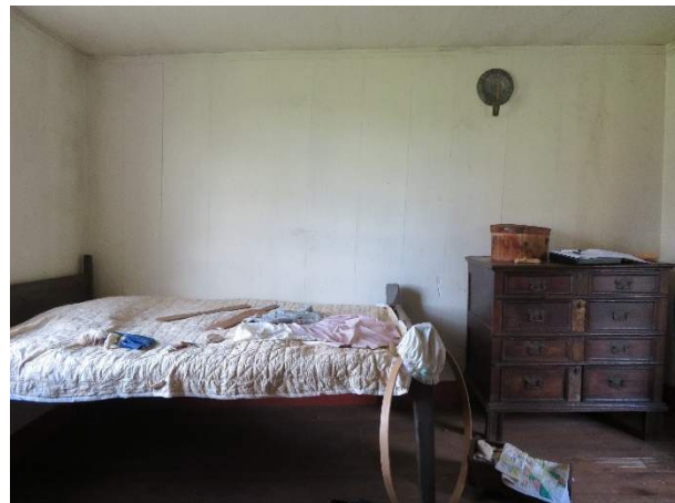
Photo 321. Room 6 (106), looking south at wall believed to be historic planks.
