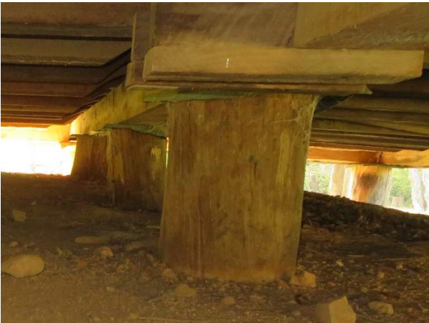
Photo 180. Pier P17, looking west.
