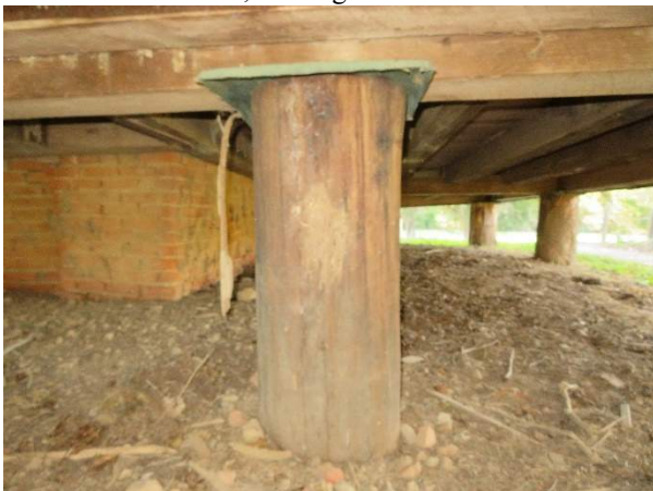
Photo 175. Pier P13, looking north.
