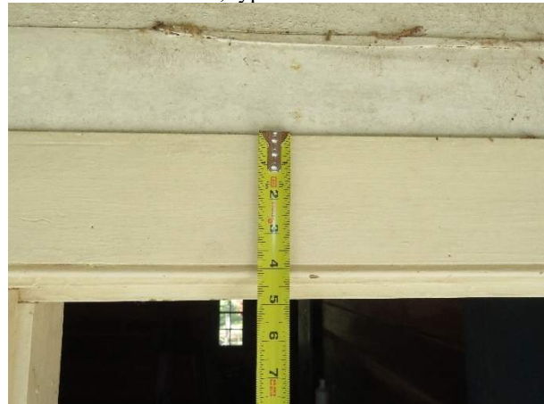
Photo 134. Head trim, typical.
