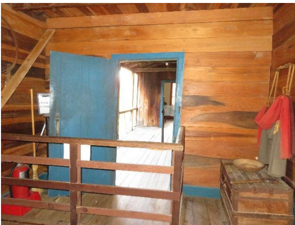
Photo 282. Door D300 from the interior.
