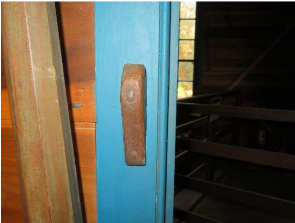
Photo 280. Latch catch on the jamb.
