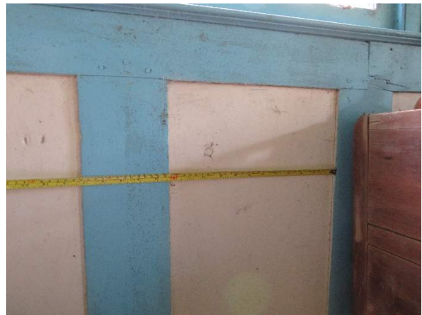
Photo 341. Typical conditions and construction of the rail-and-stile, flat panel wainscot.
