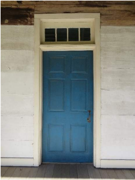
Photo 151. Door D700, overall.
