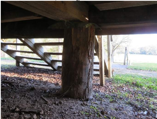
Photo 161. Pier P3, looking south.
