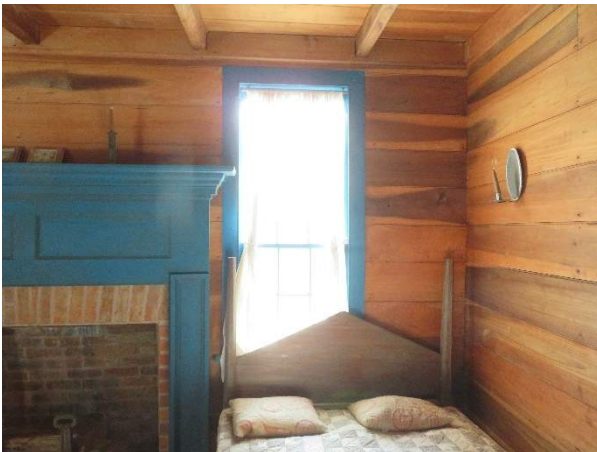
Photo 250. Window W201 from the interior.
