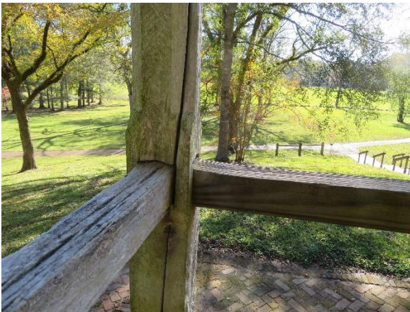
Photo 40. Checking of south gallery post through the railing connection.
