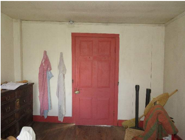
Photo 286. Door D600 from the interior.
