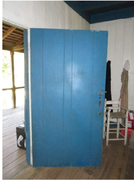
Photo 125. Door D101, from interior with door open.
