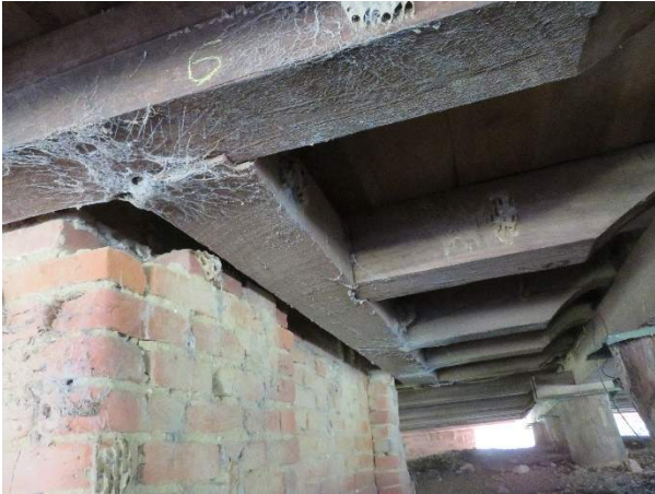
Photo 205. Floor framing system on north side of central chimney.
