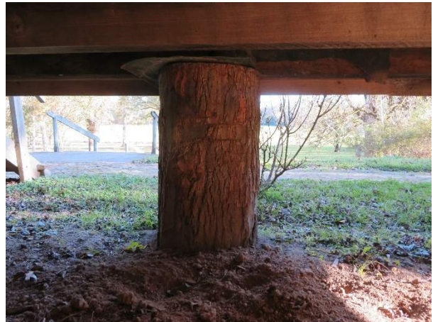
Photo 160. Pier P2, looking south.
