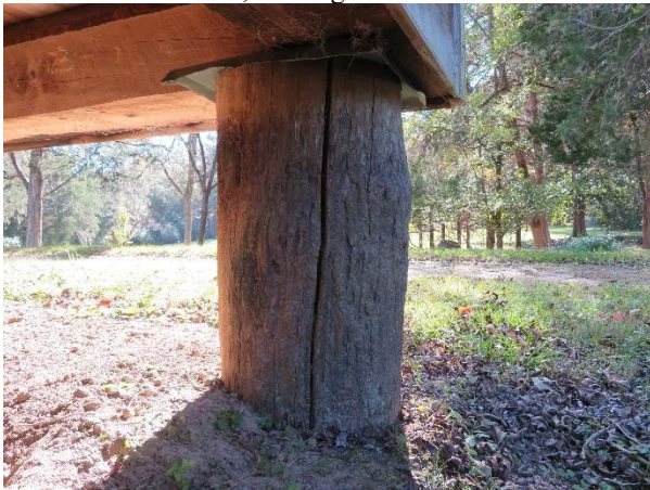
Photo 185. Pier P22 at northwest corner.
