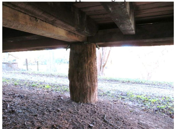
Photo 176. Pier P14, looking east.
