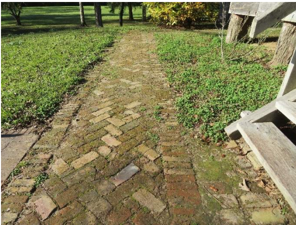
Photo 13. Brick paver walkway at the south side of the house.
