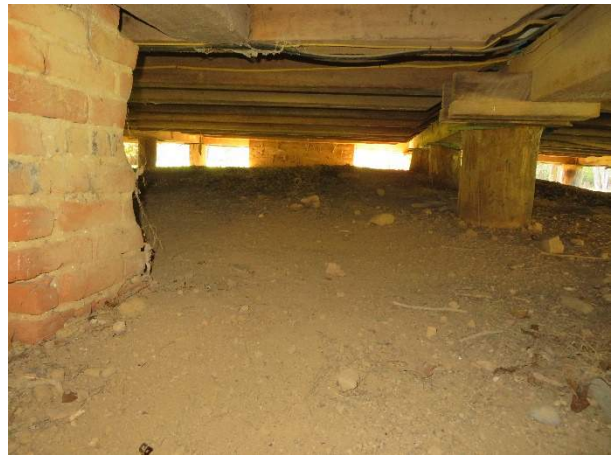
Photo 202. High point of crawlspace under Room 3 (103), looking west.
