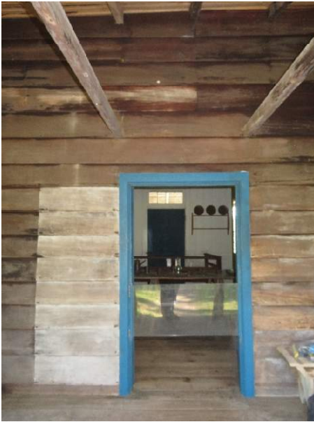
Photo 124. Door D101. overall, looking south.
