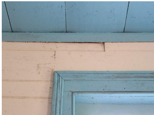
Photo 266. Head and jamb trim were in good condition.
