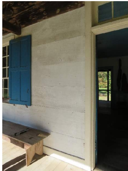
Photo 58. Board siding on south elevation.
