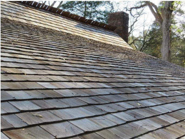
Photo 49. Wood shake roofing at north roof slope.
