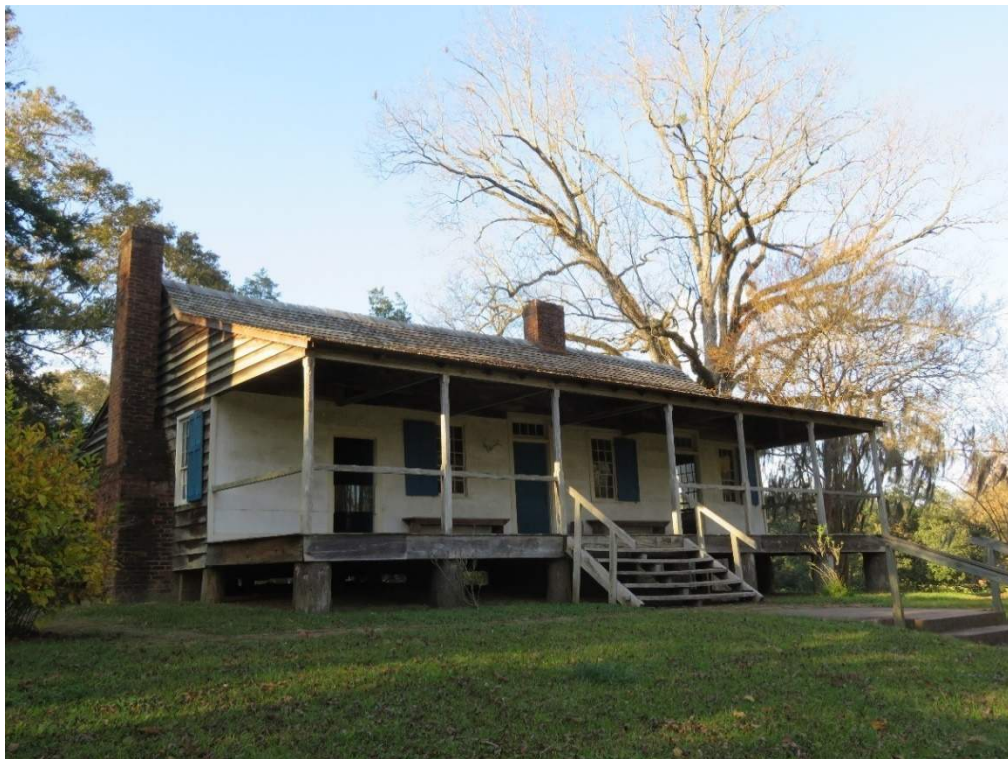
Photo 2. Main (south) elevation from the south.
