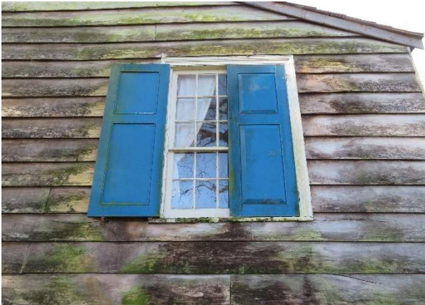
Photo 102. Window W601, overall.
