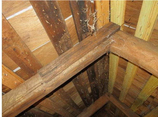
Photo 224. Repair to the scarf joint at the apex of Rafter Bay R2.
