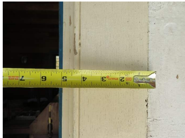
Photo 132. Jamb trim, typical.
