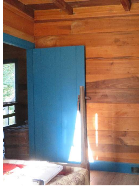
Photo 136. Door D201, looking east.
