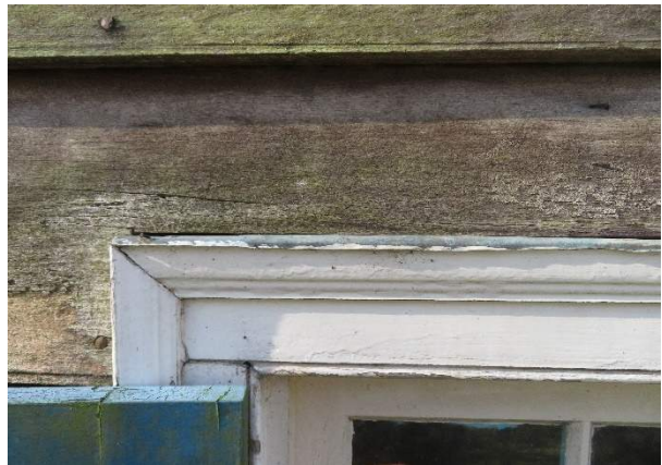
Photo 119. Sheet metal flashing cap at window head.
