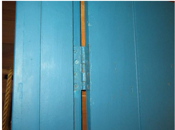
Photo 281. Butt hinges for Door D201.
