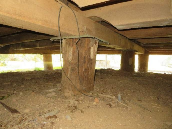
Photo 182. Pier P19, looking northeast.
