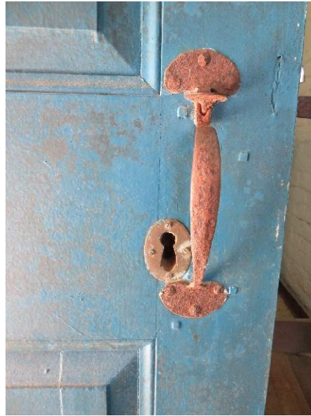
Photo 152. Exterior door hardware.
