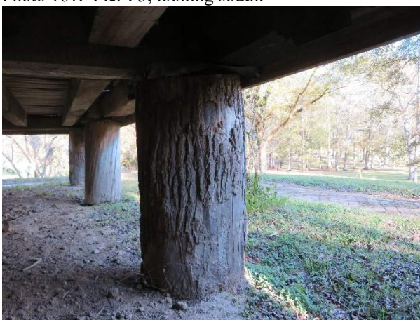
Photo 163. Pier P5, looking southeast.
