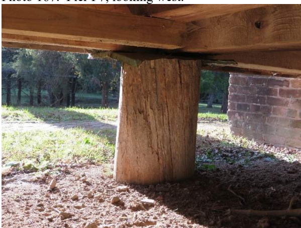
Photo 169. Pier P8, looking west.
