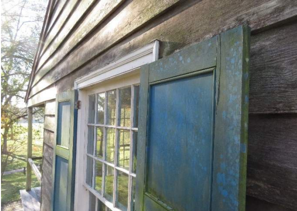
Photo 114. Window W701, top of window looking south.
