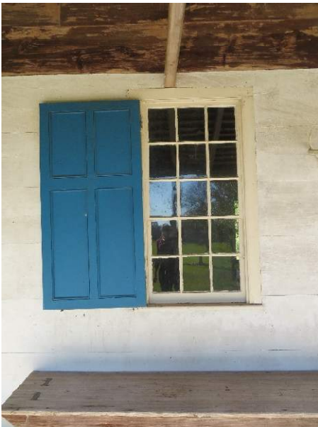
Photo 81. Window W100, overall.
