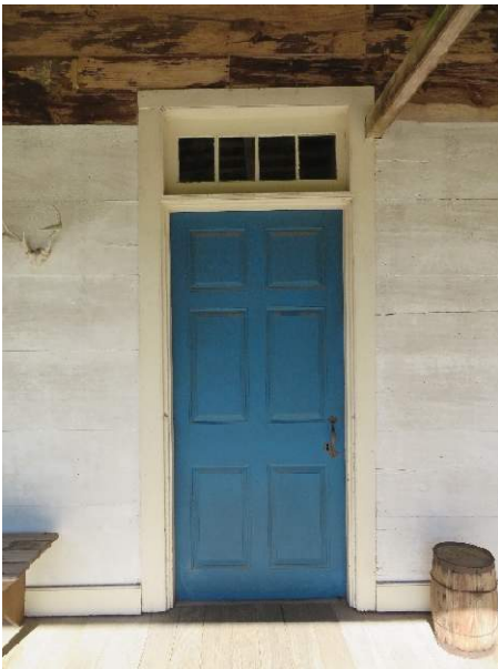
Photo 120. Door D100, overall.
