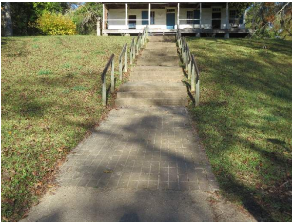
Photo 9. Main stairs, looking north to house.
