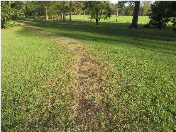
Photo 8. Paved walkway from main walk to the grape arbor, showing deteriorated and uneven paving.
