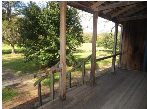
Photo 45. North gallery posts.
