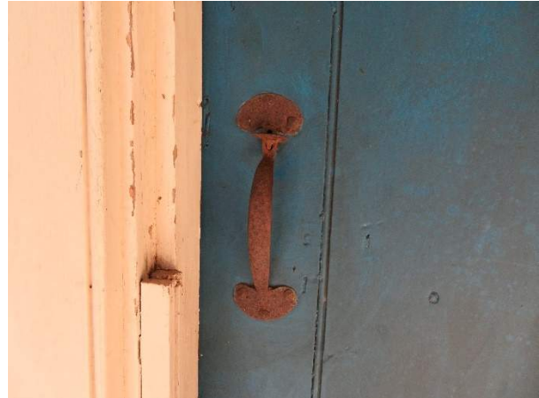
Photo 130. Exterior door hardware.
