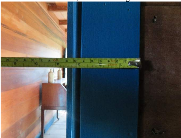
Photo 137. Door jamb, typical.
