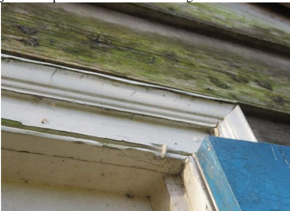
Photo 106. Sheet metal flashing cap at window head.
