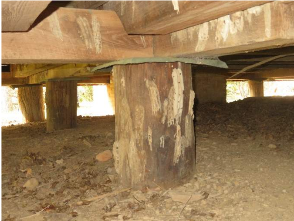
Photo 171. Pier P10, looking west.
