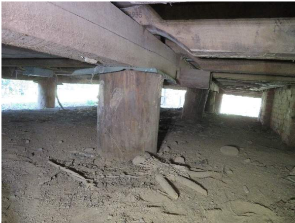
Photo 183. Pier P20, looking south.
