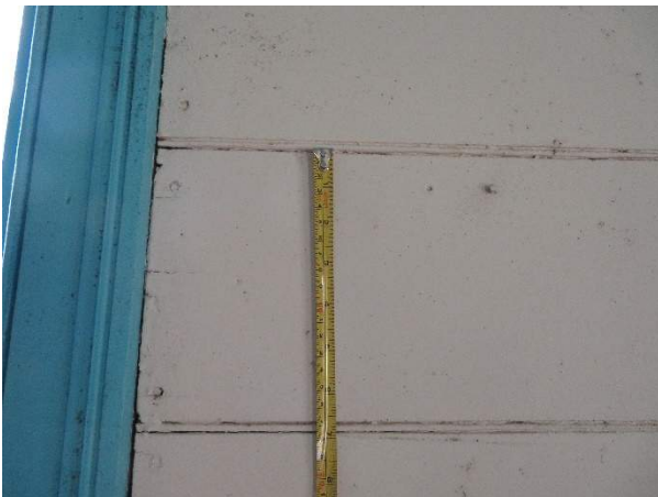
Photo 334. Typical horizontal wall board.
