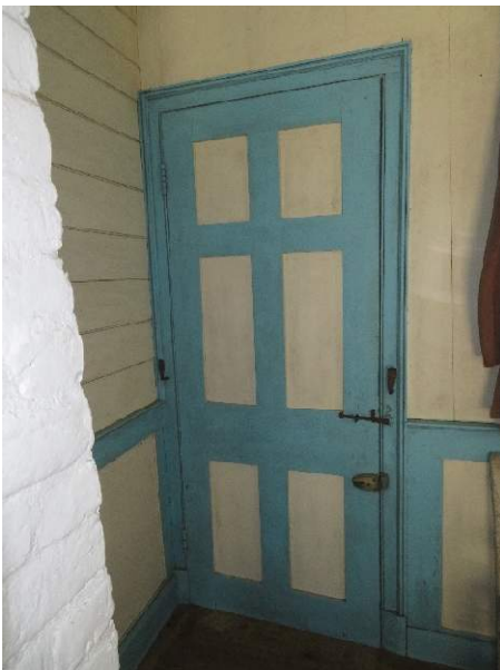
Photo 292. Door D701 from the interior.
