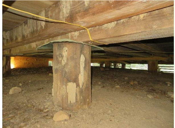
Photo 172. Pier P11, looking west.
