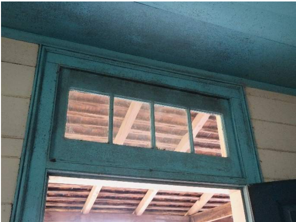
Photo 291. Transom of Door D700.
