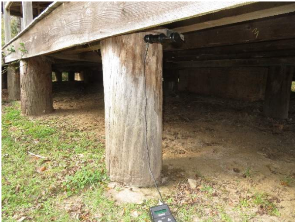
Photo 165. Pier P6, looking northwest.
