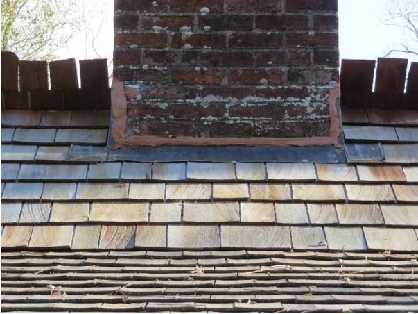
Photo 52. Flashing and sealant at chimney.
