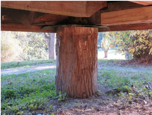
Photo 159. Pier P1, looking southwest.
