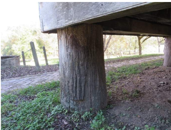
Photo 199. Pier P29 at northeast corner.
