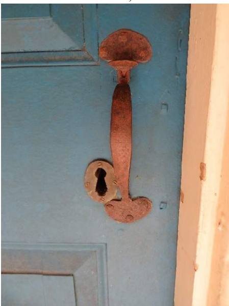
Photo 122. Exterior hardware of Door D100.
