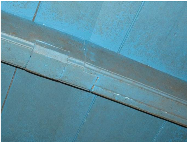
Photo 304. Mid-span splice at the first ceiling beam from the west.
