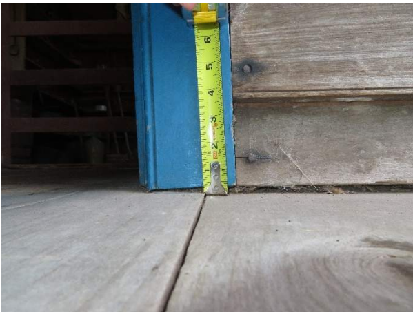
Photo 143. Change in slope at door threshold.
