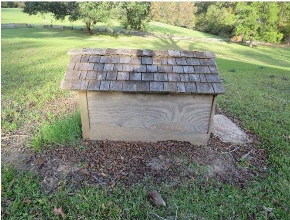
Photo 21. Wood shed over fire hydrant.
