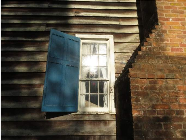
Photo 95. Window W201, overall.
