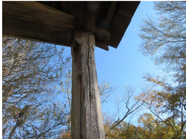
Photo 39. Checking of south gallery posts.
