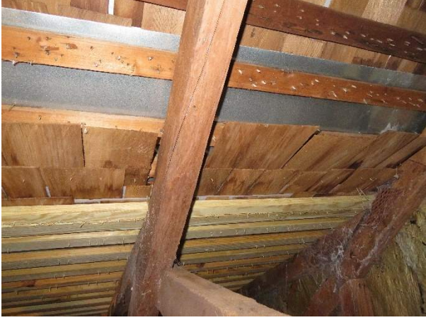
Photo 53. Sheet metal flashing at change in roof slope.
