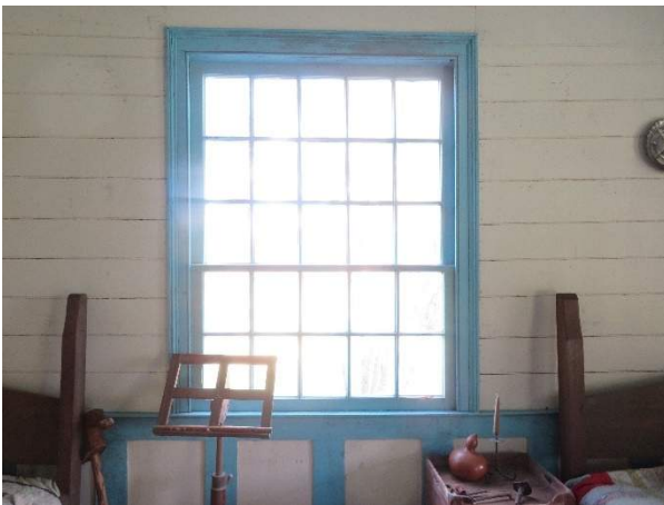
Photo 265. Window 701 from the interior.
