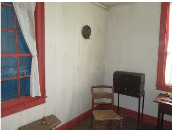
Photo 324. Wall boards in the northeast corner.
