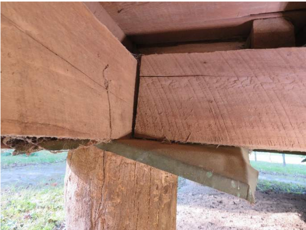
Photo 178. Copper cap flashing at the head of Pier P15.
