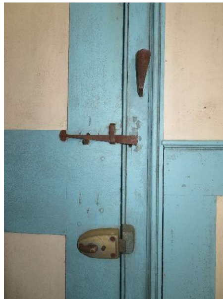
Photo 293. Interior hardware, showing the lift-latch and brass rim lock.
