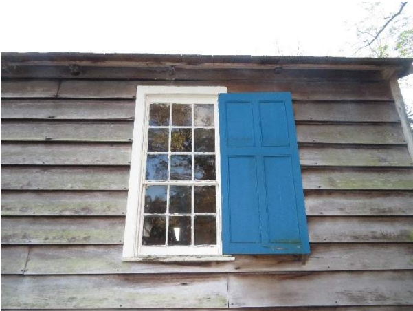
Photo 99. Window W300, overall.
