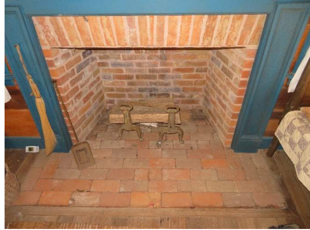
Photo 76. Fireplace and brick hearth in Room 2 (102).
