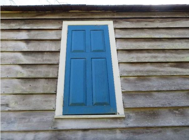
Photo 100. Window W600, overall.
