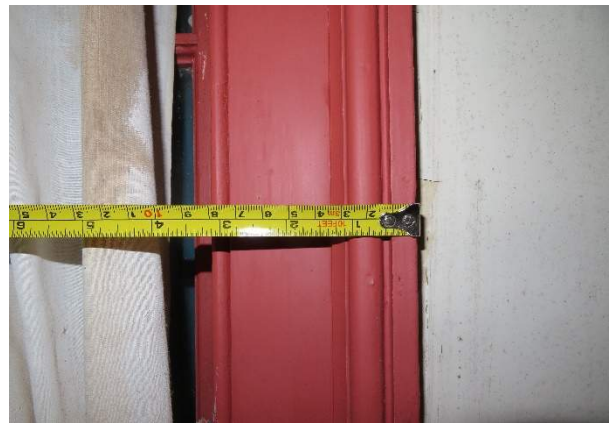
Photo 255. Jamb trim at Window W600 was in good condition.
