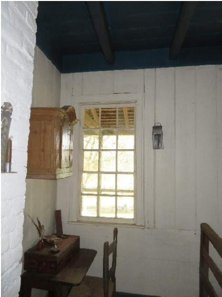
Photo 244. Window W101 from the interior.
