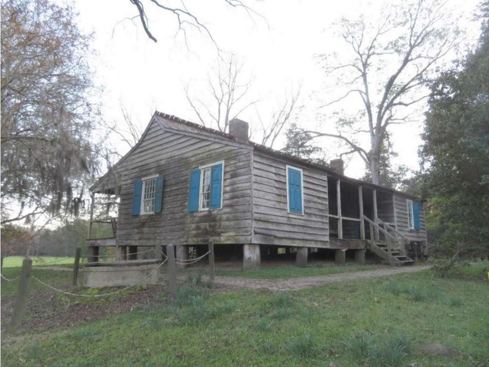
Photo 4. East and rear (north) elevations, from the northeast.
