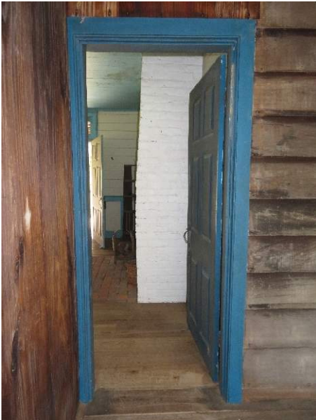
Photo 155. Door D701, looking south.
