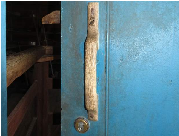
Photo 141. Exterior door hardware.
