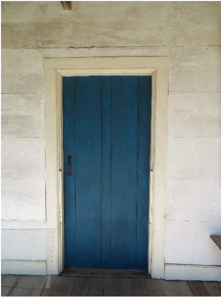
Photo 129. Door D200, overall.
