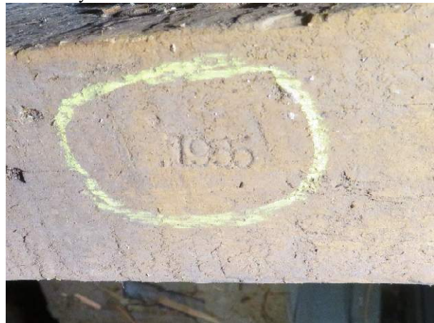
Photo 226. "1955" identifying brand on the collar tie for Rafter Bay R7.
