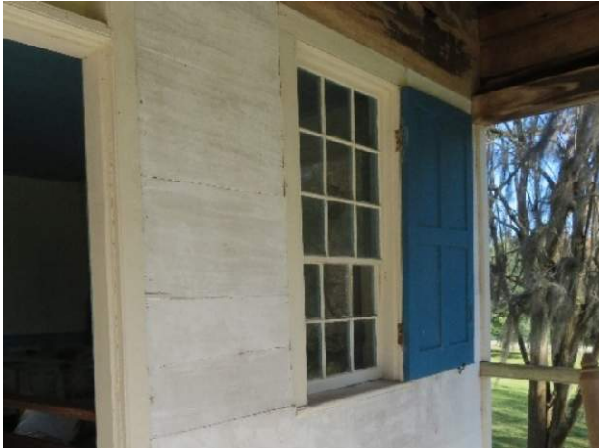
Photo 108. Window W700, overall.
