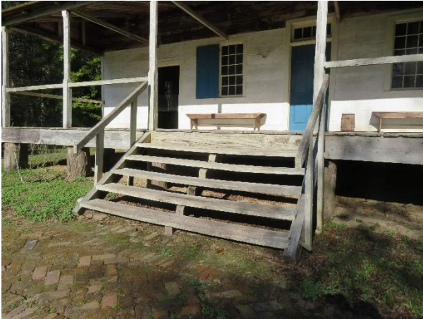
Photo 31. Exterior stairs to south gallery.
