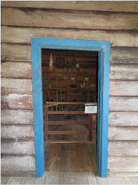
Photo 139. Door D300, overall.
