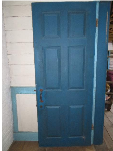
Photo 156. Door D701, looking east.
