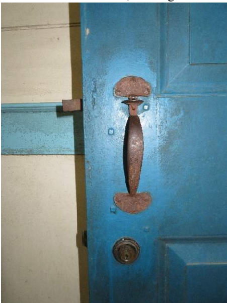
Photo 157. Exterior door hardware.
