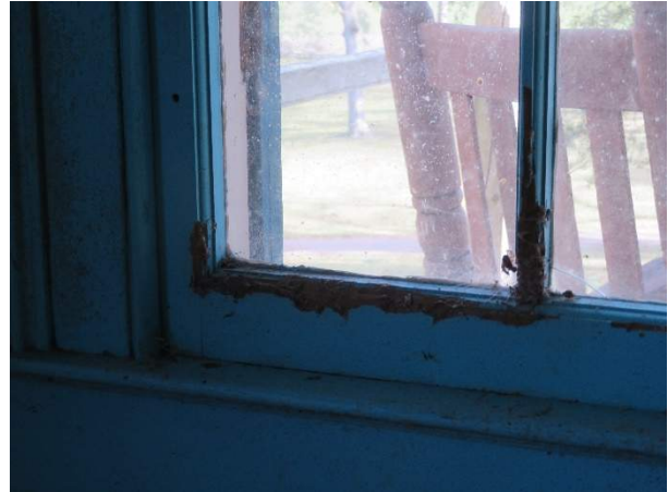
Photo 264. Patch repairs to the interior of the lower sash.
