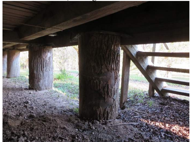
Photo 162. Pier P4, looking southeast.
