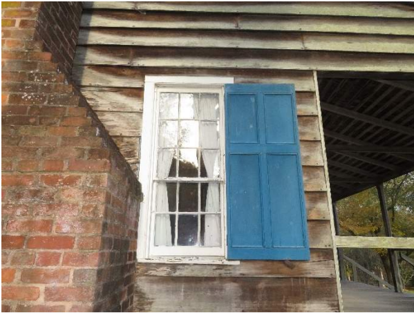
Photo 89. Window W200, overall.
