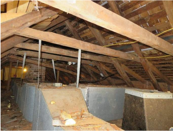
Photo 221. View in attic looking west.
