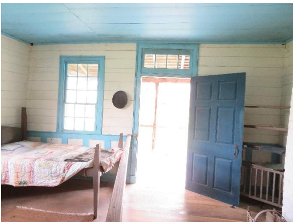
Photo 289. Door D700 from the interior.
