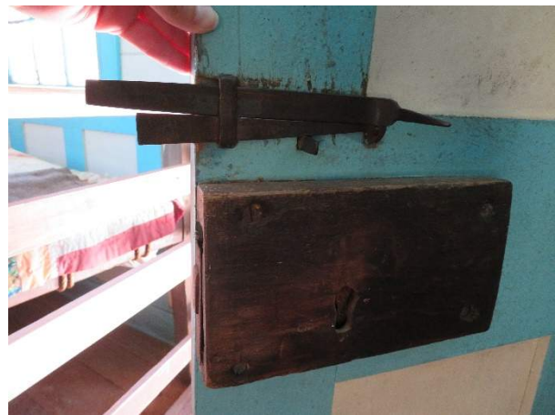
Photo 290. Rim lock and lift-latch on the interior of Door D700.
