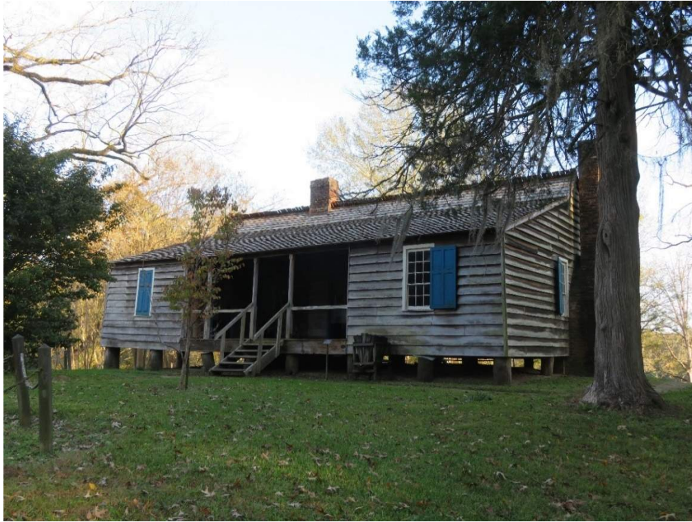
Photo 5. Rear (north) elevation, from slightly northwest.
