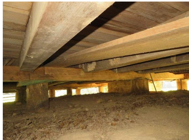
Photo 204. Floor framing system below Room 3 (103), looking southwest showing joists running north-south.
