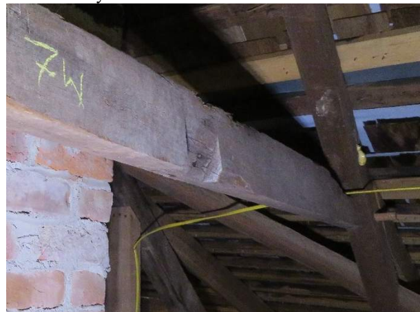
Photo 232. Repurposed timber used as a collar tie in rafter Bay R11.
