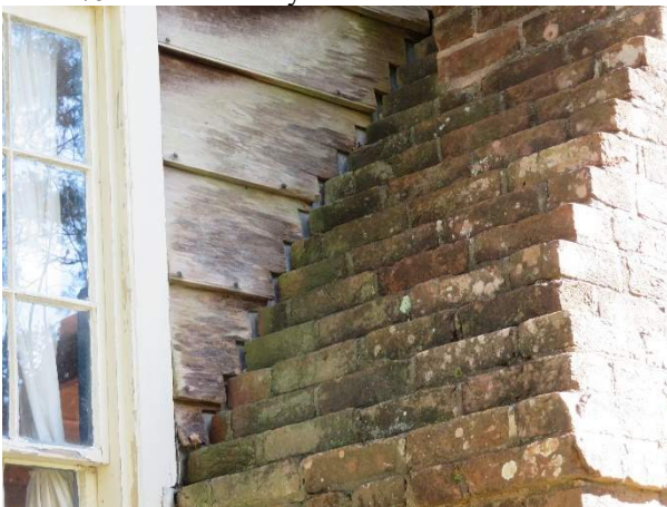
Photo 77. Step flashing behind bricks and siding at west chimney.
