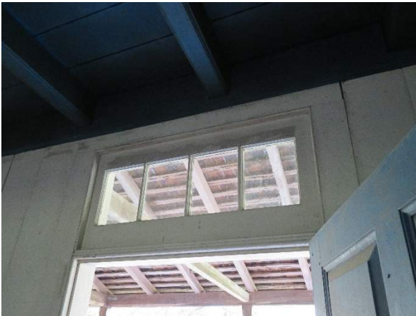
Photo 271. The transom of Door D100.
