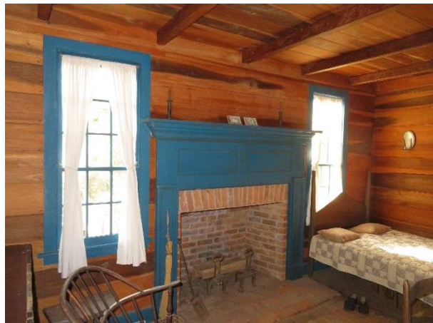
Photo 313. Fireplace mantel on the west wall.
