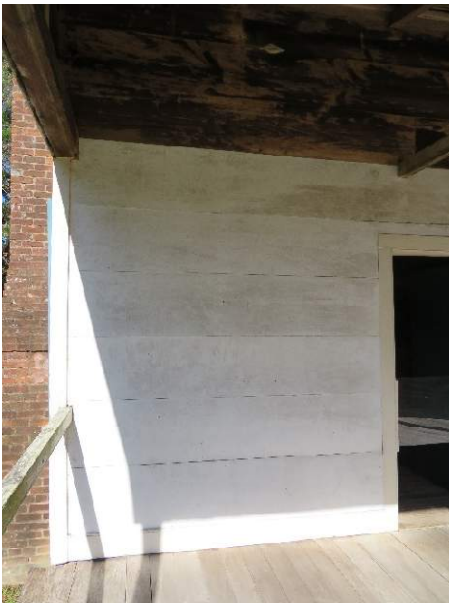
Photo 57. Board siding on south elevation.
