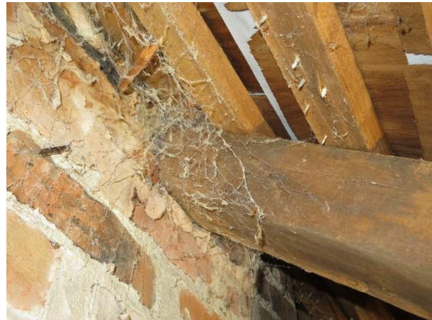
Photo 234. Primary rafter bearing at brick masonry chimney in Rafter Bay R12.
