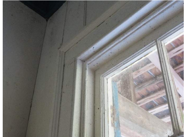
Photo 245. Jamb and head trim were in good condition.
