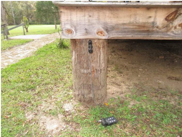
Photo 167. Pier P7, looking west.
