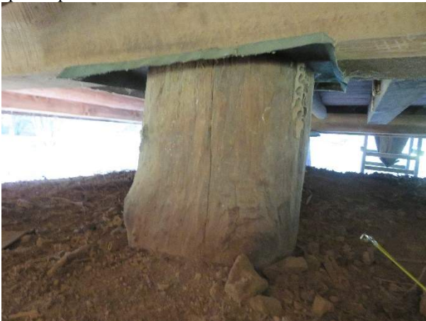
Photo 179. Pier P16, looking north.
