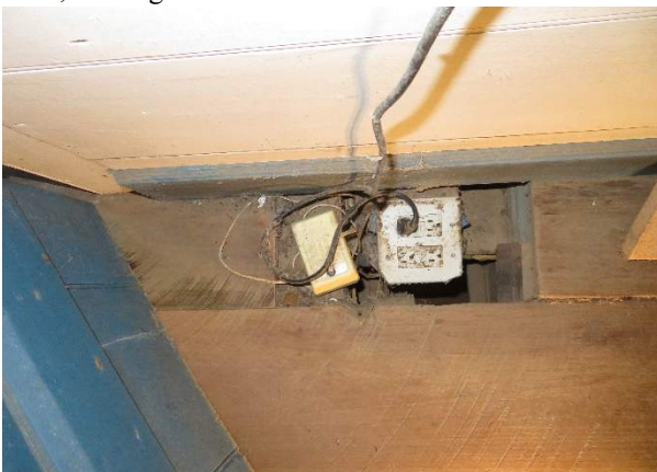
Photo 298. Hole cut in the flooring for electrical service.
