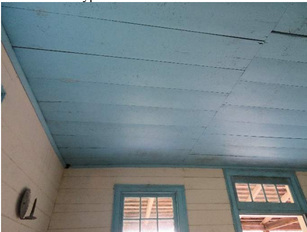
Photo 336. Ceiling boards in the southeast corner of the room.
