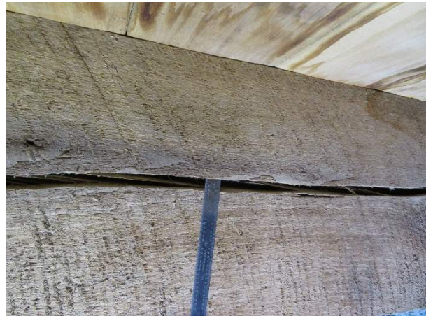
Photo 212. Checking at Joist J4.
