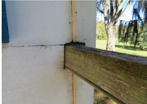
Photo 56. East rail connection at board siding and corner trim.
