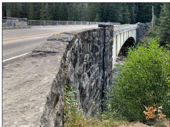
Native stone on Fryingspan Creek Bridge and its abutments
