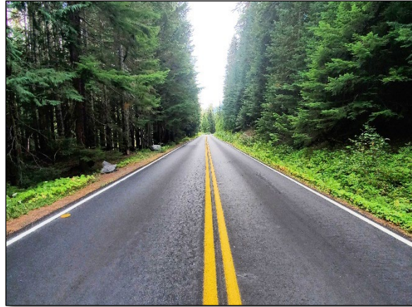
The narrow road corridor of the Yakima Park Highway within the project area
