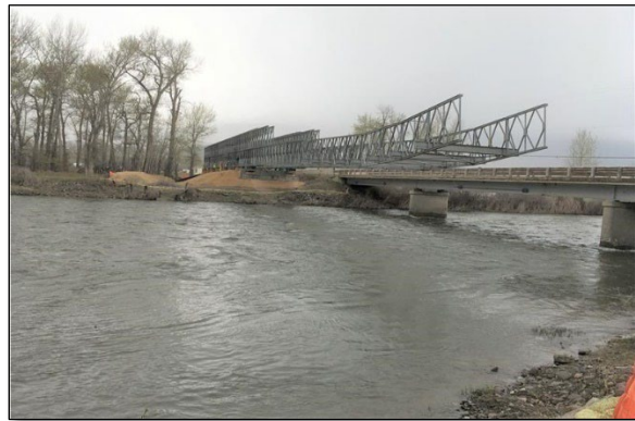
A portion of a temporary prefabricated bridge (FHWA photo)
