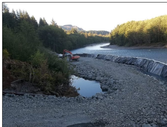
Example dewatered work zone area (FHWA photo)
