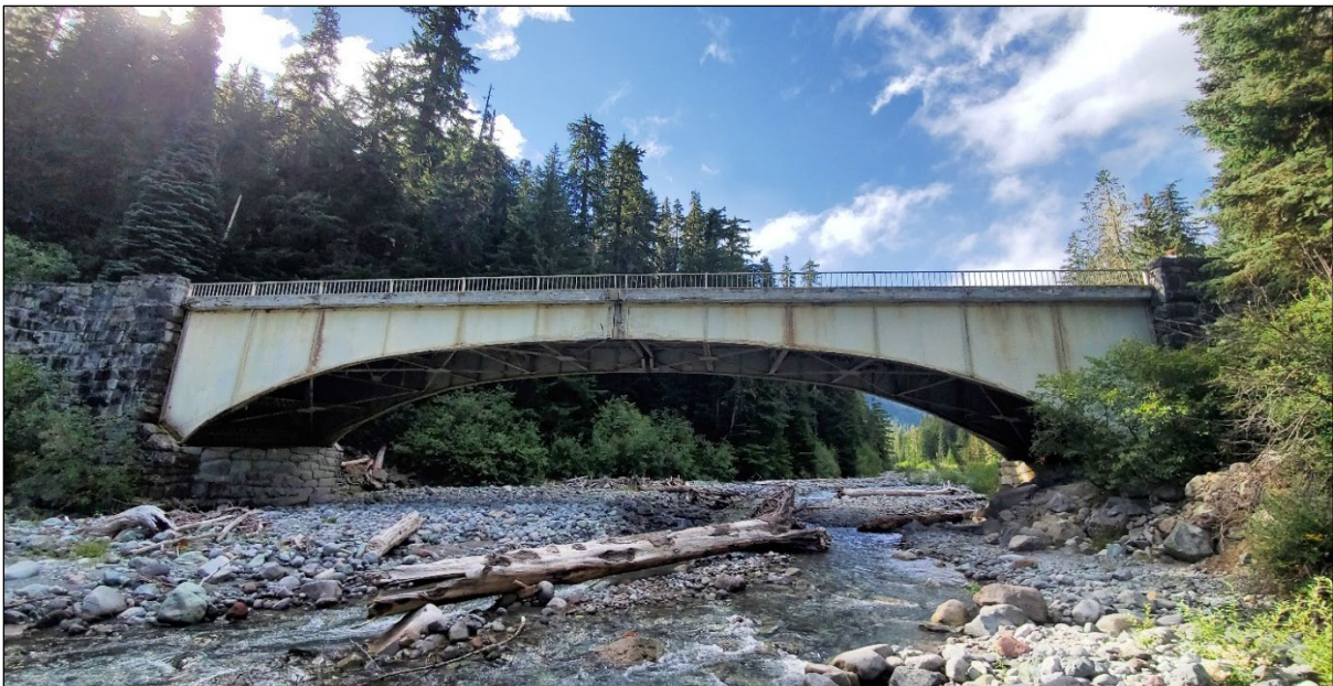
Fryingspan Creek Bridge, NPS photograph 2021
