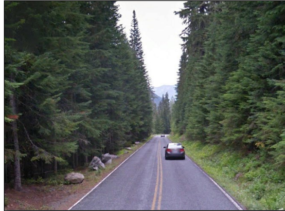
Rock barriers along the Yakima Park Highway within the project area (Google Earth)
