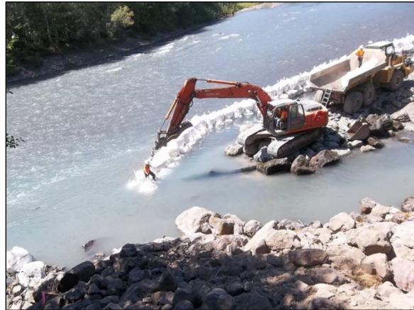
Supersack berm installation for in-water work (FHWA photo)
