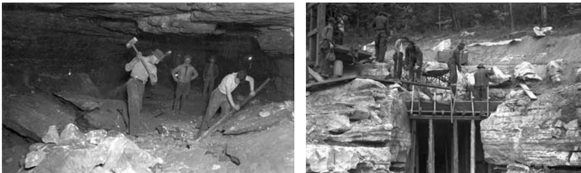
**FIGURE 1-1.** Two examples of cave modifications made by the Civilian Conservation Corps. Left is a photograph of trail building in the Historic Section, 1935; right, construction of the Frozen Niagara Entrance, 1938. (NPS images from Western Kentucky University, <http://www.wku.edu/Library/nps/ccc>).
