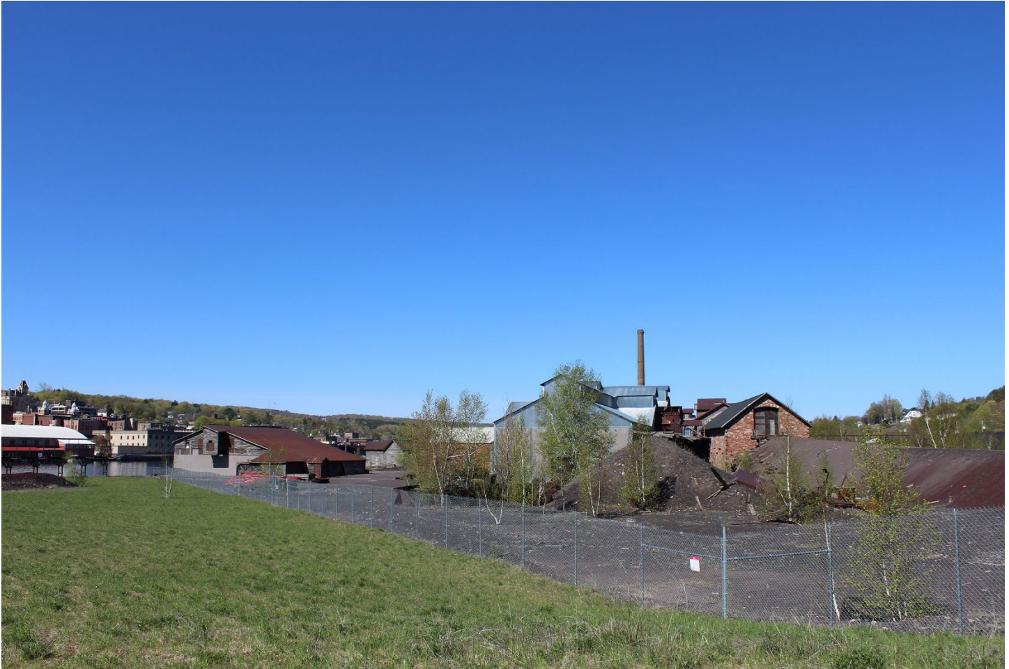
Quincy Smelting Works Landscape Character Area 4. Left to right: Dockside Warehouse (MAP ID# 178), Assay Office (MAP ID# 176), Scale House (MAP ID# 177), Casting Plant (MAP ID# 171), East Slag Pile and Steel Trestle, and Mineral House (MAP ID# 169). Boiler Stack (MAP ID# 156) in background.
