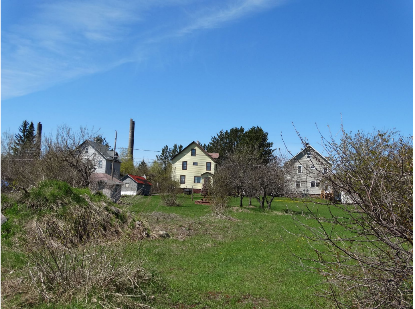
Lower Pewabic Housing Location Landscape Character Area 3. Back of residences along West Lower Pewabic Street (left to right: MAP ID#s 132, 133 and 134). The No. 6 and No. 2 Boiler House Stacks (MAP ID# 026 and 025) in the distance, left.
