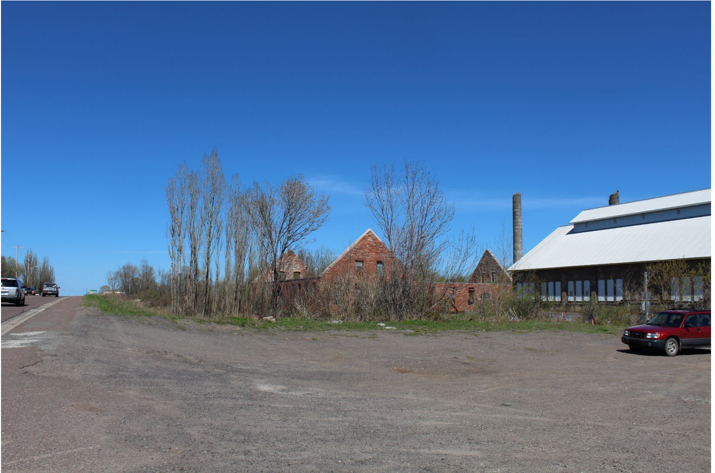
Quincy Mine Industrial Core Landscape Character Area 1. Quincy Blacksmith Shop Ruin (MAP ID# 24) and Quincy Machine Shop (MAP ID# 023). US-41 at extreme left.
