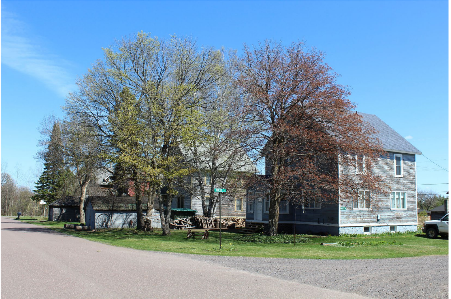
Lower Pewabic Housing Location Landscape Character Area 3. Residences along West Lower Pewabic Street (right to left: MAP ID#s 138, 139, 140 and 141).
