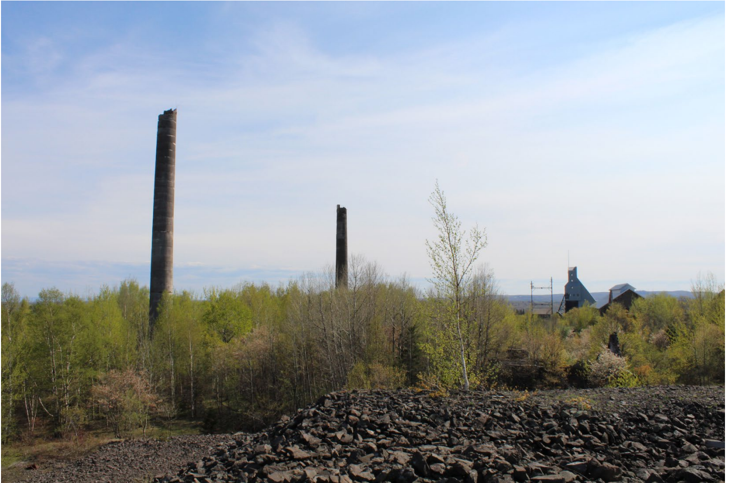
Quincy Mine Industrial Core Landscape Character Area 1. Poor rock pile in the No. 6 area; the No. 6 Boiler House Stack (MAP ID#26), and the No. 2 Boiler House Stack (Map ID# 025) on the left. The roof of the Quincy Machine Shop (MAP ID# 023) and the No. 2 Shaft-Rockhouse (Map ID# 006) are in the distance.
