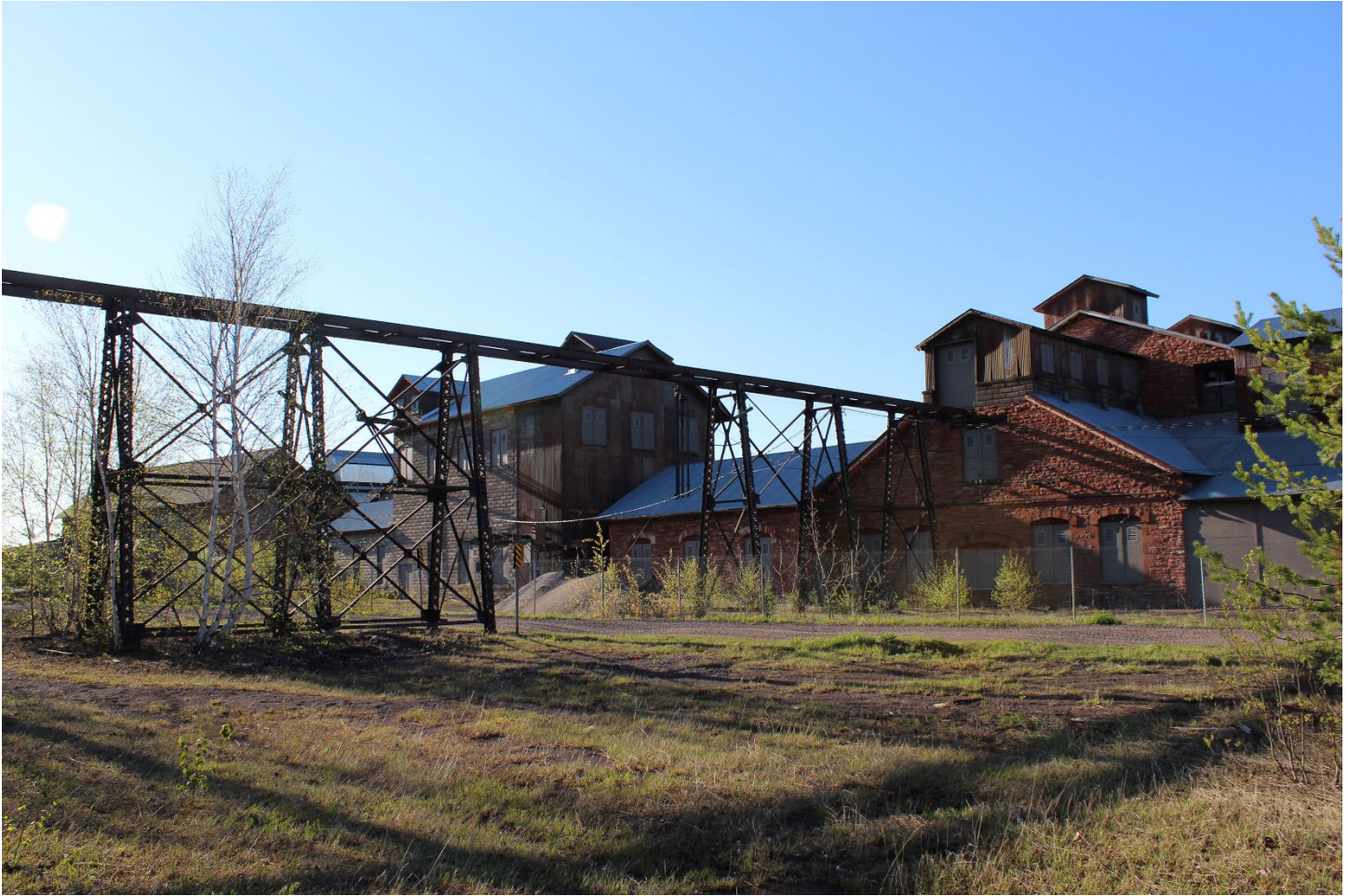
Quincy Smelting Works Landscape Character Area 4. Steel Trestle (MAP ID# 151) in foreground; right to left: Cupola Furnace Building (MAP ID# 159), Pump House Addition (MAP ID# 162), Crushing Plant (MAP ID# 163), Briquetting Plant (MAP ID# 165) and Mineral House (MAP ID# 169).
