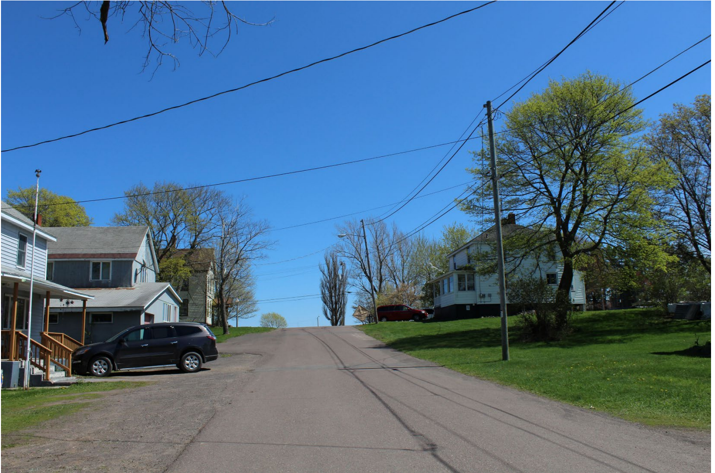
Quincy Hill Housing and Mine Management Landscape Character Area 2. Limerick Housing Location, residences along 5 th Street (left to right: MAP ID#s 117 porch, 116, 115, 114).
