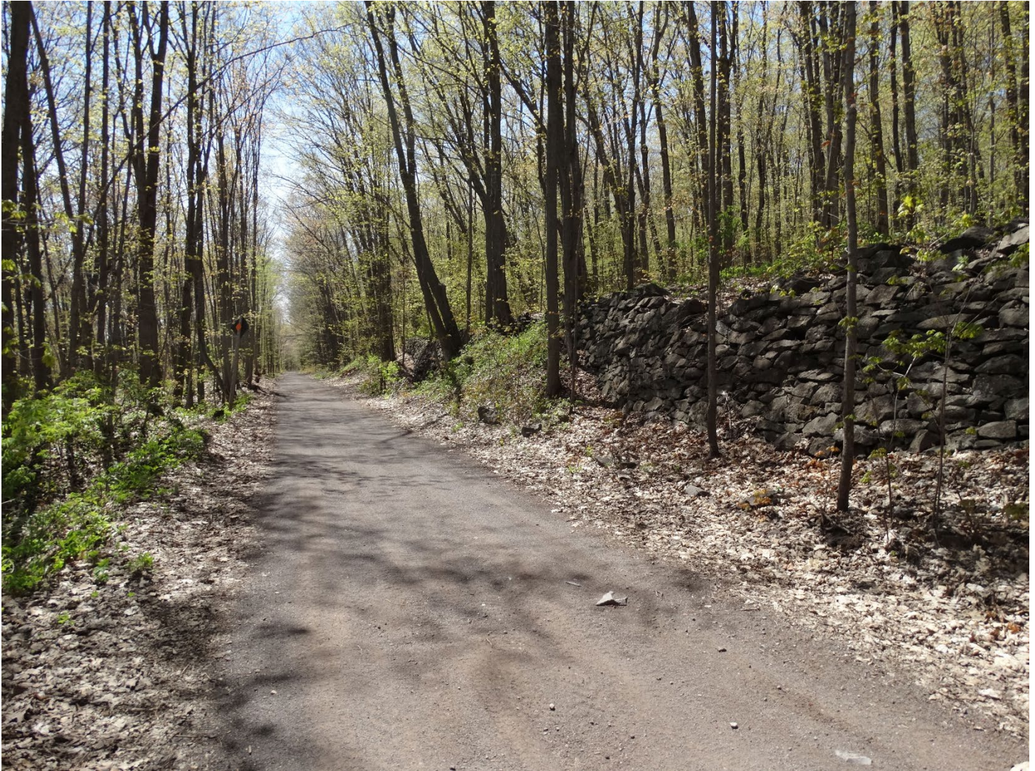
Quincy and Torch Lake Railroad Corridor, Landscape Character Area 6. A typical view along the corridor, with a stone retaining wall on the uphill side.
