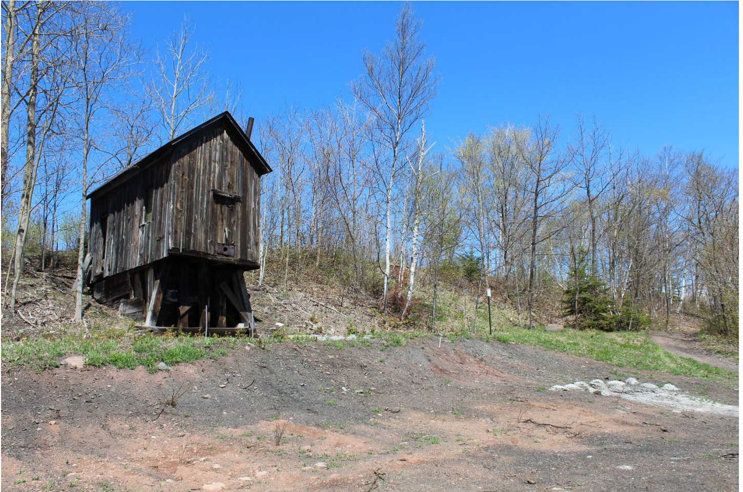
Quincy Mine Industrial Core Landscape Character Area 1. The Quincy and Torch Lake Railroad Water Tank (MAP ID# 002).
