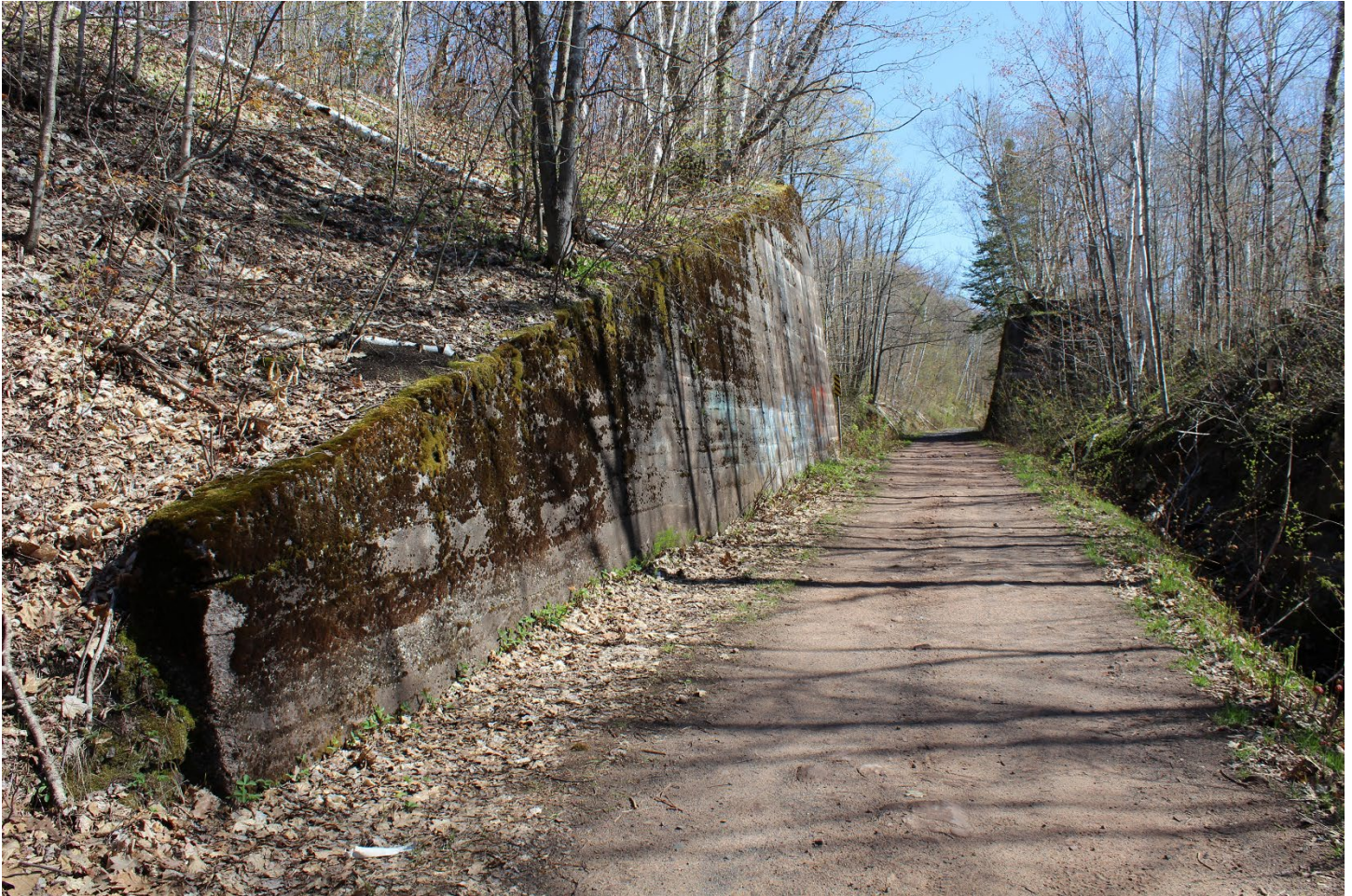
Quincy and Torch Lake Railroad Corridor, Landscape Character Area 6. Detail of retaining walls along the corridor.
