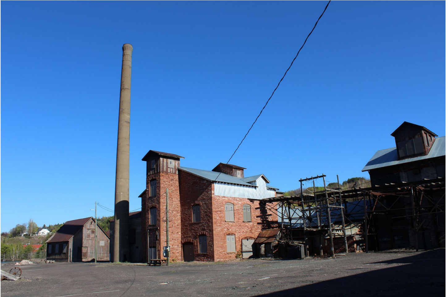
Quincy Smelting Works Landscape Character Area 4. Left to Right: Cooper Stock (MAP ID# 155), Boiler Stack (MAP ID# 156), Cupola Furnace Building (MAP ID# 159), Woodshed (MAP ID# 160), Wood and Metal Trestle (MAP ID# 161), Steel Trestle (MAP ID# 164) and Briquetting Plant (MAP ID# 165).
