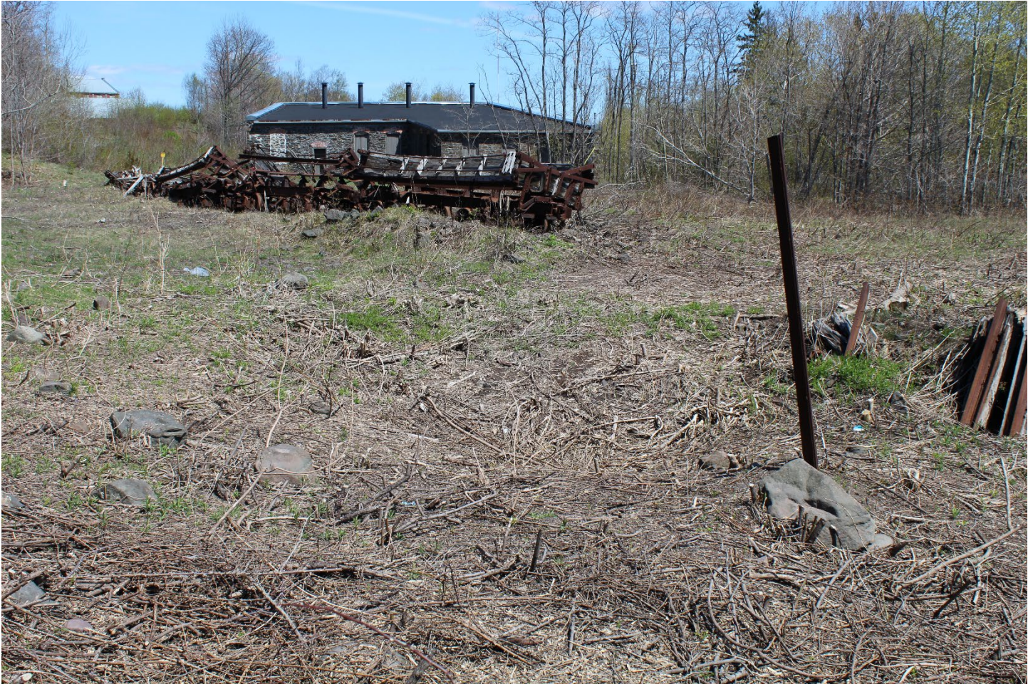
Quincy Mine Industrial Core Landscape Character Area 1. The Quincy and Torch Lake Railroad Engine House (MAP ID# 001) and remnants of rolling stock.
