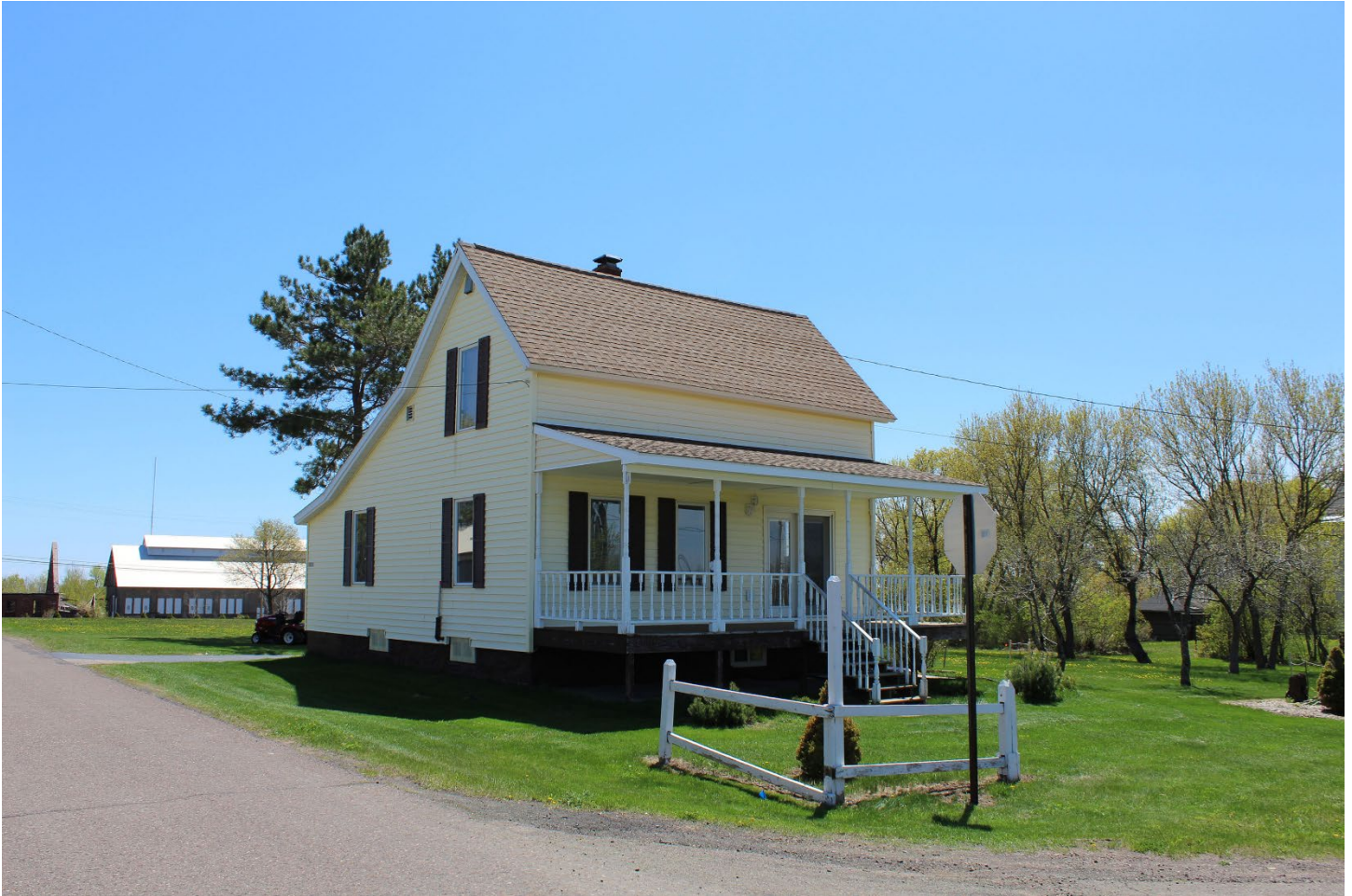
Quincy Hill Housing and Mine Management Landscape Character Area 2. Limerick Housing Location, Limerick Street residence (MAP ID# 090). The Quincy Machine Shop (MAP ID# 023) in the background.
