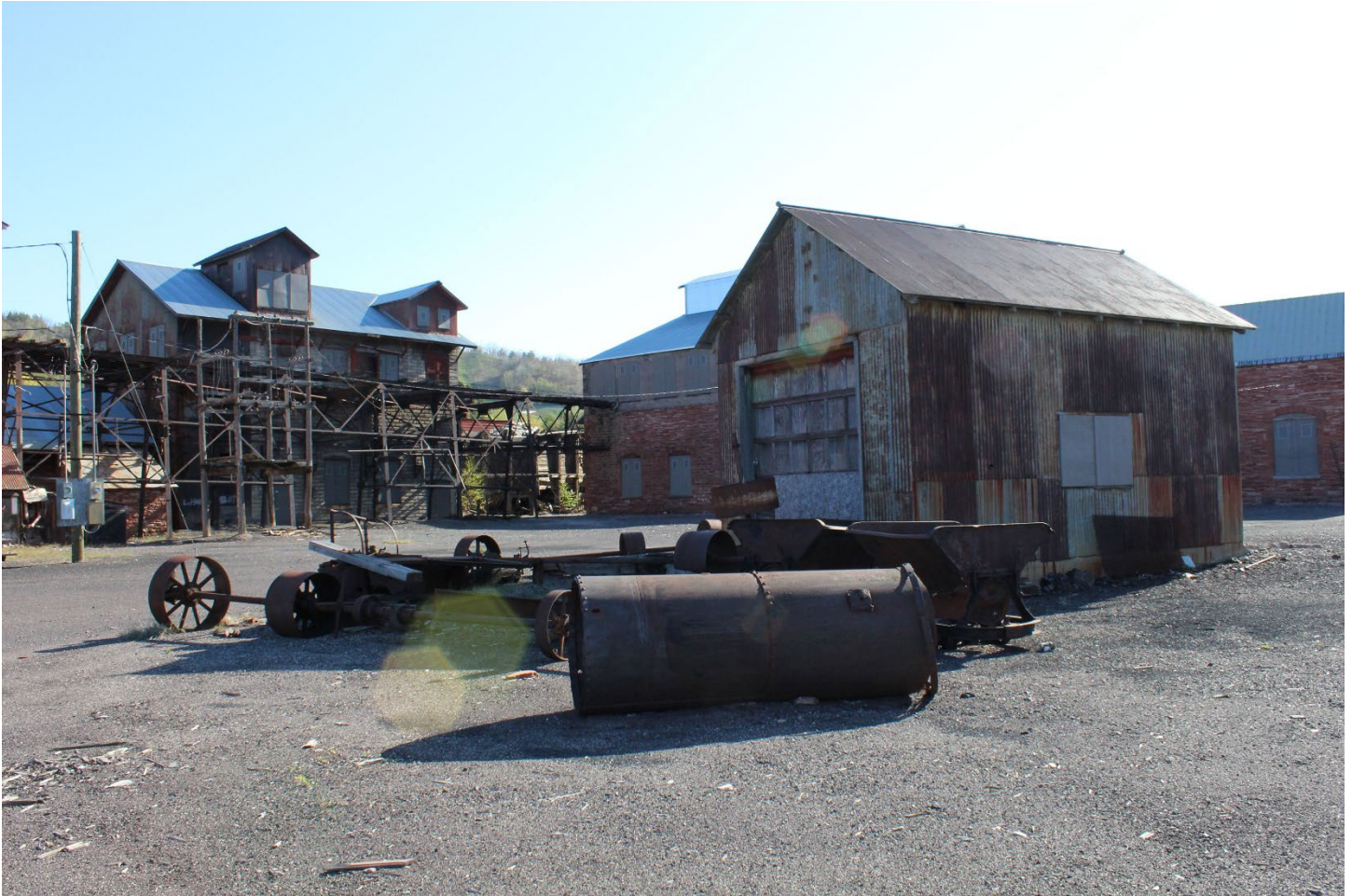
Quincy Smelting Works Landscape Character Area 4. Scale House (MAP ID# 174) in foreground. Left to right: Wood and Metal Trestle (MAP ID# 161), Steel Trestle (MAP ID# 164), Briquetting Plant (MAP ID# 165) and 1898 Reverberatory Furnace Building (MAP ID # 173)
