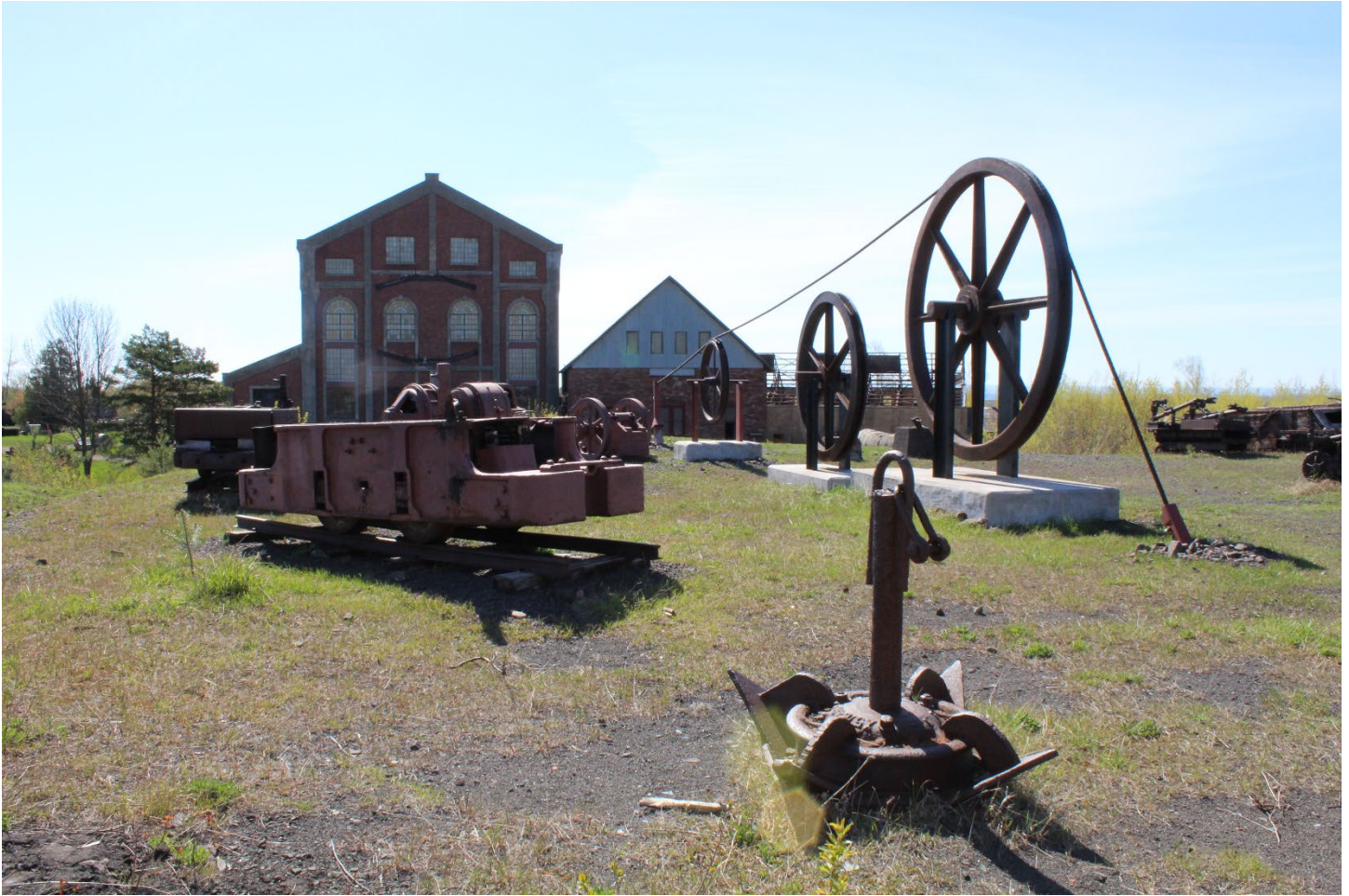
Quincy Mine Industrial Core Landscape Character Area 1. Left to right: the 1918-1920 No. 2 Hoist House (MAP ID# 012), the 1894-1985 No. 2 Hoist House (MAP ID# 013) and three pulleys (MAP ID# 011).
