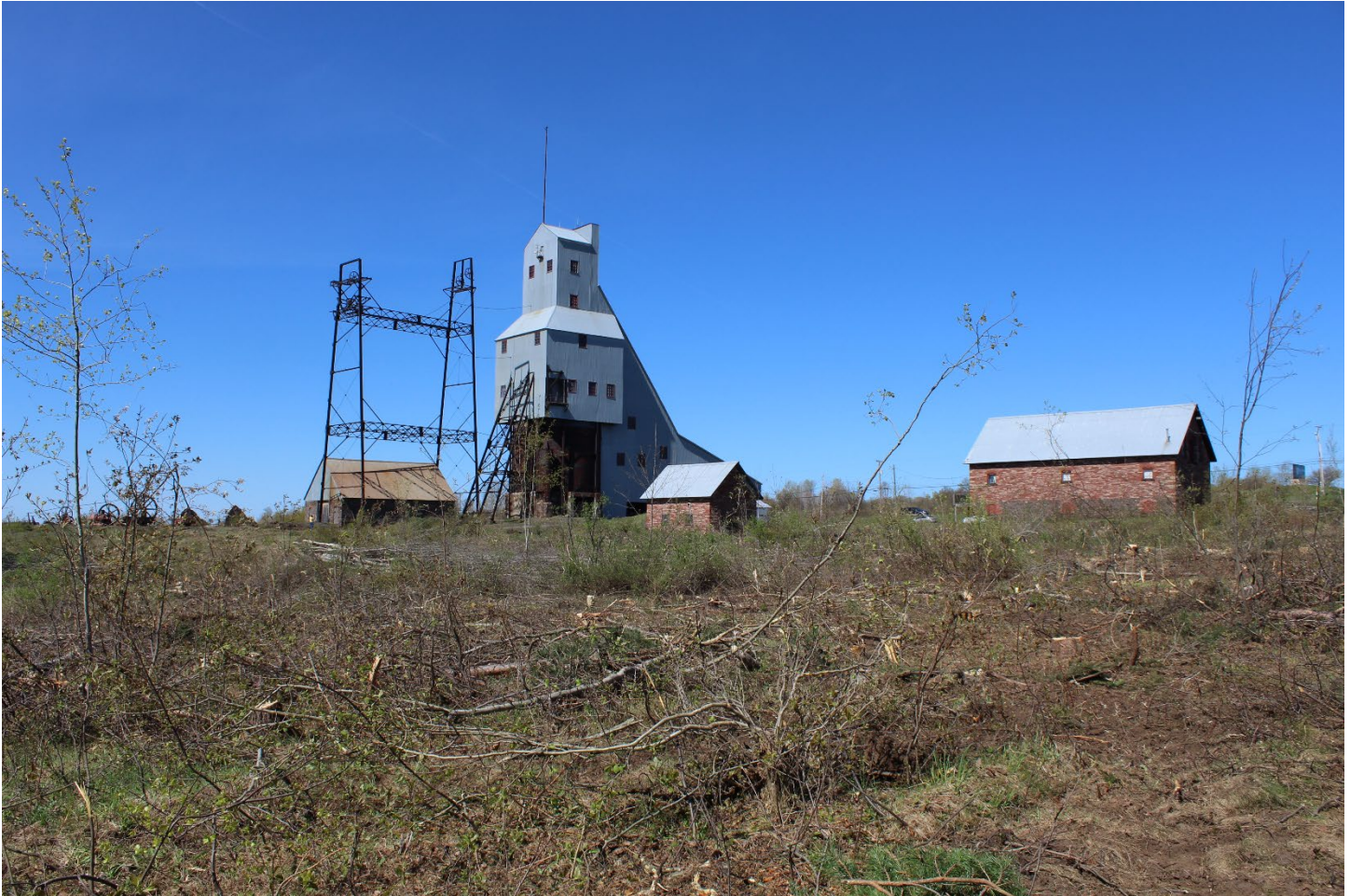
Quincy Mine Industrial Core Landscape Character Area 1. Left to right: the 1882 No. 2 Hoist House (Map ID# 008), Pulley Stand (MAP ID# 007), the No. 2 Shaft-Rockhouse (Map ID# 006), Oil House (MAP ID# 010) and Supply Office (MAP ID# 009).
