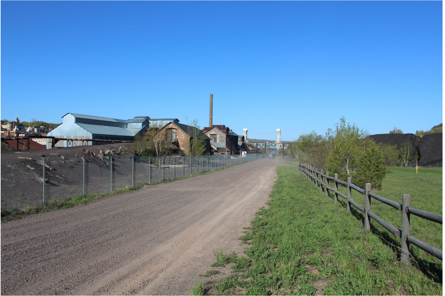
Quincy Smelting Works Landscape Character Area 4. East Slag Pile and Steel Trestle (MAP ID# 170) in left foreground. Left to Right: Casting Plant (MAP ID# 171), Mineral House (MAP ID# 169), Briquetting Plant (MAP ID# 165) and North Slag Pile (MAP ID# 151). Boiler Stack (MAP ID# 156) in background.
