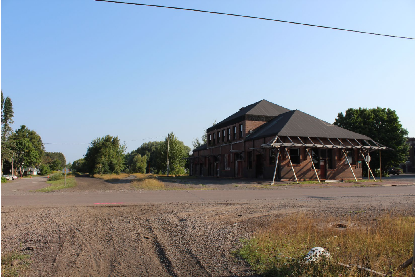
Village of Calumet Housing Location Landscape Character Area F, Mineral Range Railroad Depot (Map ID# 349) and adjacent rail corridor.
