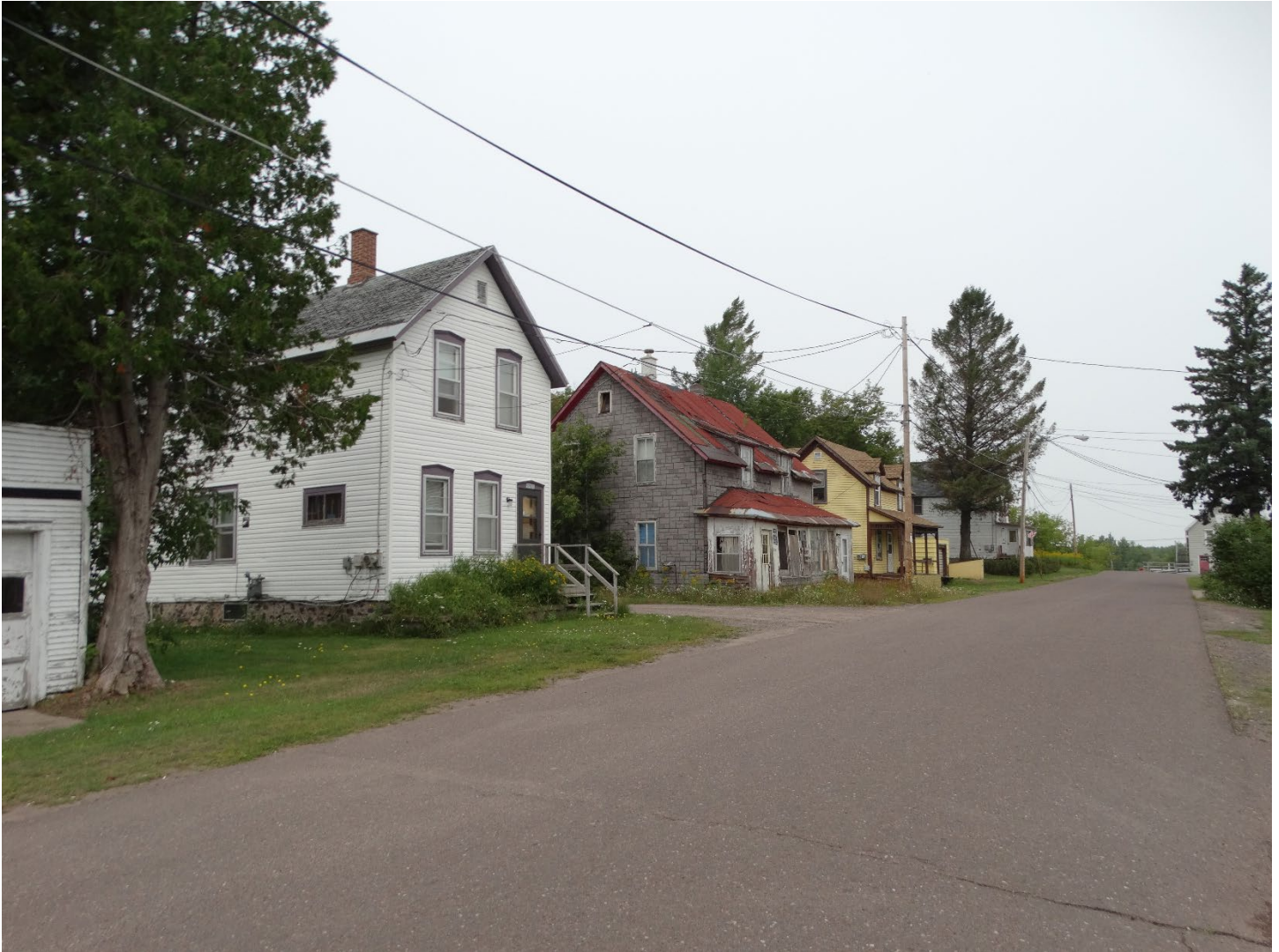
Blue Jacket Housing Location Landscape Character Area E. Worker housing along Fourth Street (left to right: Map ID#s 240, 242, and 241).
