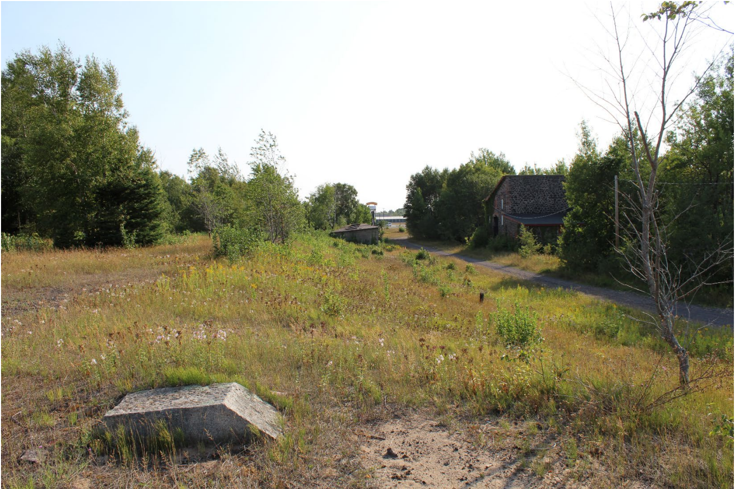
Calumet and Hecla Mine Industrial and Management Core Landscape Character Area A. The C&H Pattern Storage Warehouse (Map ID# 60) is on the right, the Sand Storage Building (Map ID# 59) in the middle, and railroad corridor to the left.
