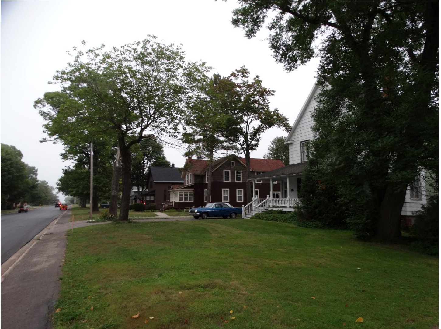
Calumet Housing Location in Landscape Character Area B. Upper-level manager housing along Calumet Avenue (right to left: Map ID#s 65, 66, and 67).
