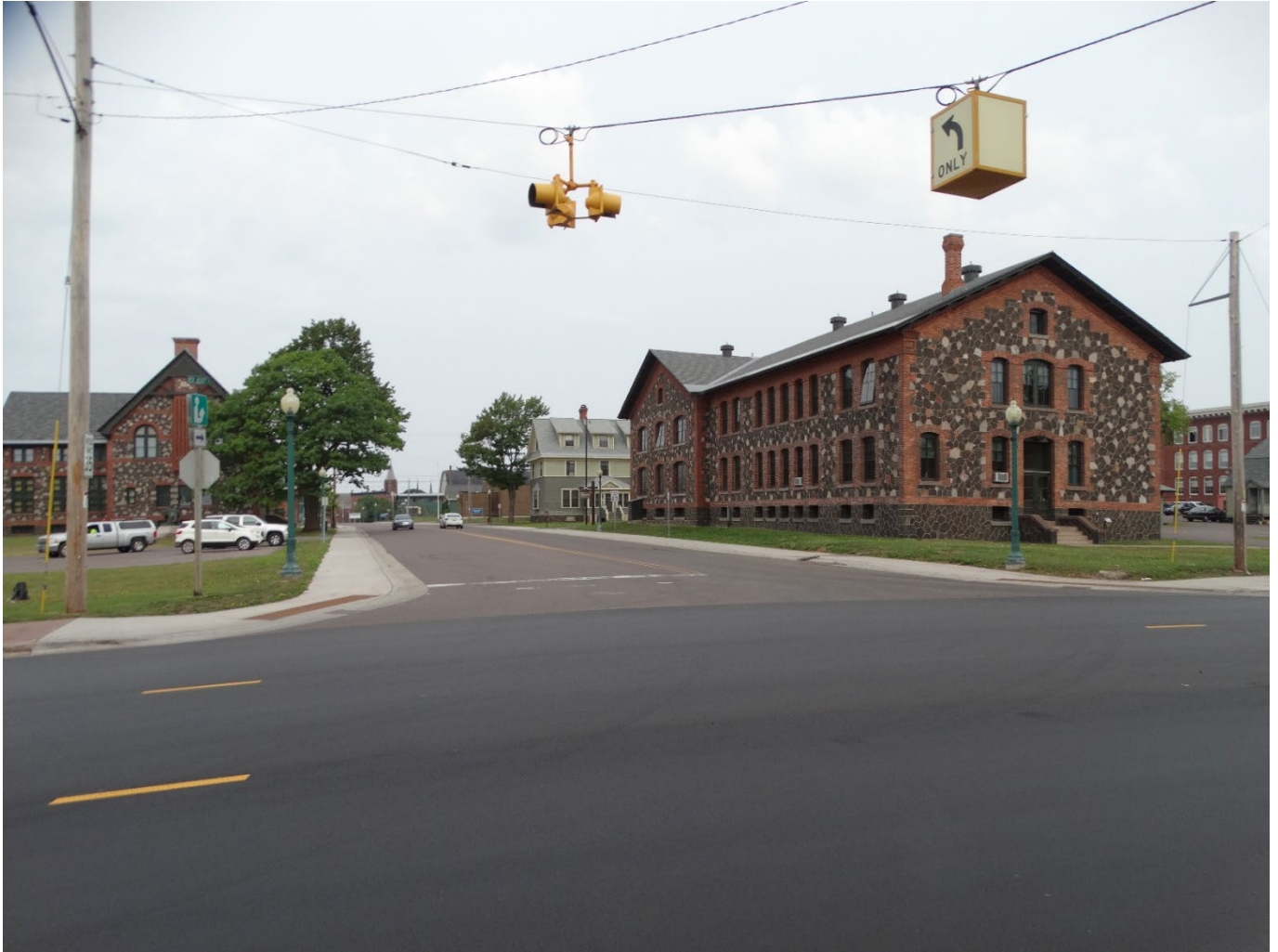
Calumet and Hecla Mine Industrial and Management Core Landscape Character Area A. The C&H Library (Keweenaw History Center, Map ID# 46) is on the left side of Red Jacket Road, the C&H General Office (Keweenaw National Historical Park Headquarters, Map ID# 47) on the right.
