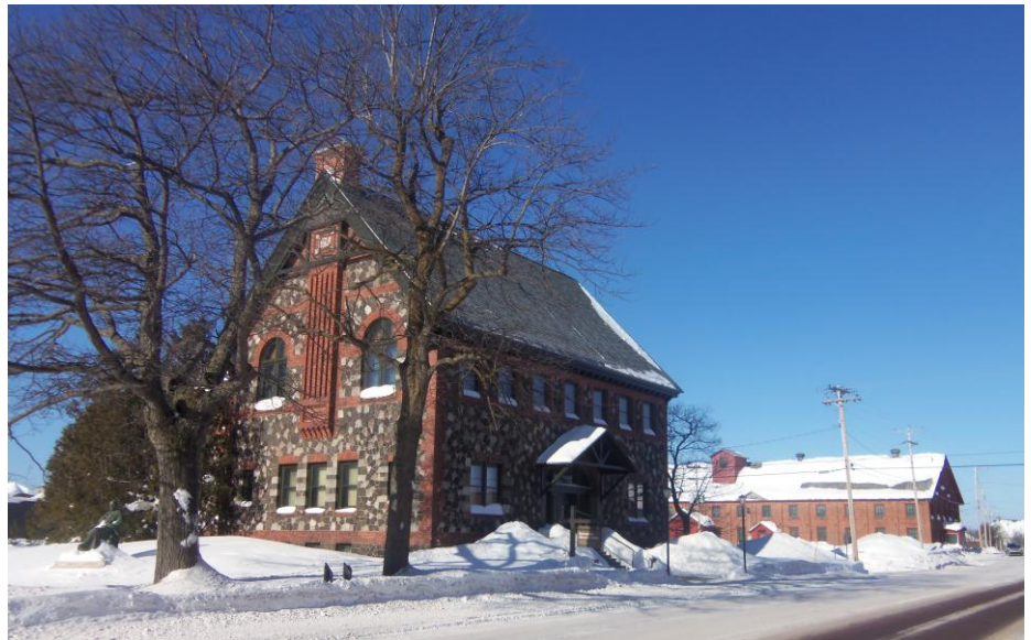
Lake Superior Collection Management Center archives and museum storage facilities, the historic former Calumet and Hecla Mining Company public library and warehouse buildings, are shown here in March of 2015 at Keweenaw National Historical Park in Calumet.
