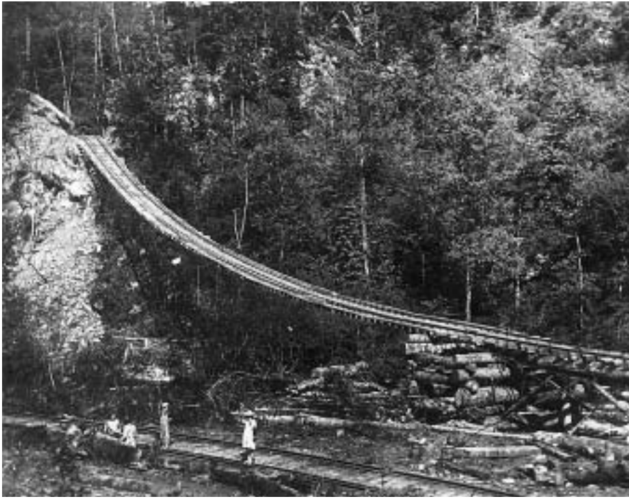
A swinging railroad bridge at the mouth of Meigs Creek swings across the Little River. These portable bridges were used to lower cars loaded with logs down the mountain.
