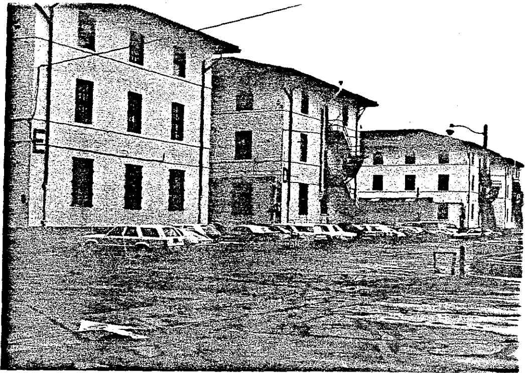
3. The four permanent army storehouses at the San Francisco Port of Embarkation in lower Fort Mason.
