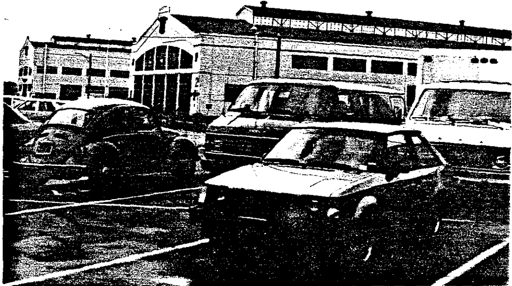
4. Piers 1, on left, and 2, San Francisco Ports of Embarkation. The shed on Pier 2 is the original, permanent shed. Pier 1's shed was reconstructed in the 1930s.
