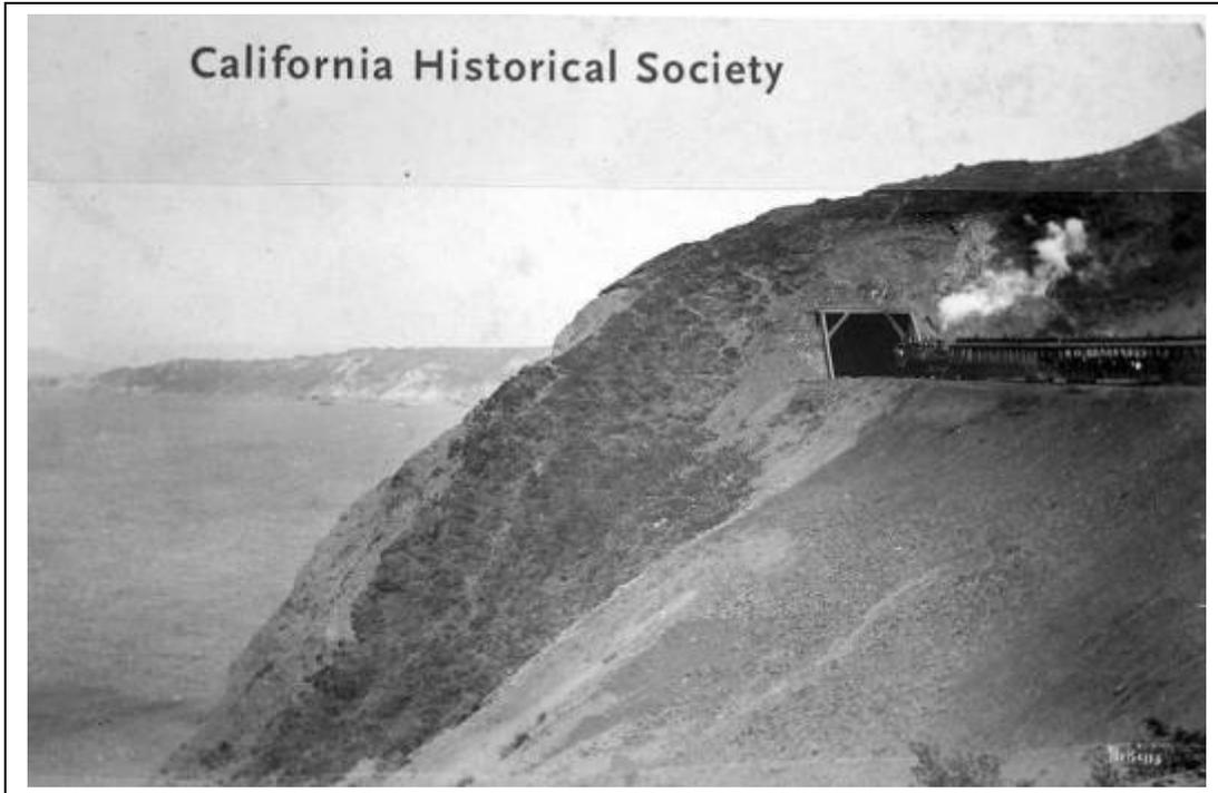
*Figure 12. Train entering the east tunnel circa 1888. This tunnel was removed shortly after. Note the freshly-graded slope below the train. (California Historical Society)*
