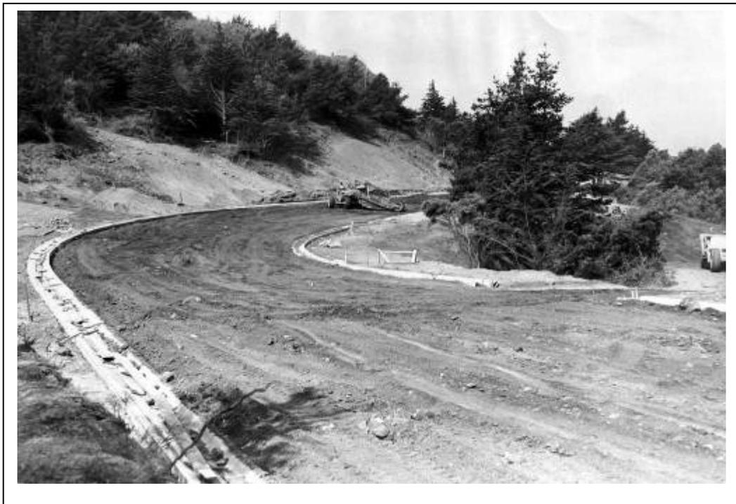
**Figure 73.** Reconstruction work on El Camino Del Mar below Fort Miley, May 17, 1951. New drainage swales are visible along both sides of the graded roadbed. (SF Public Library AAB-3499)
