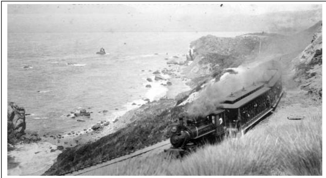
*Figure 15. Outbound train passing Helmet Rock circa 1895. Erosion has undermined the rails and ties on the outer set of tracks. Compare the tracks to those in Figure 14. (California Historical Society)*
