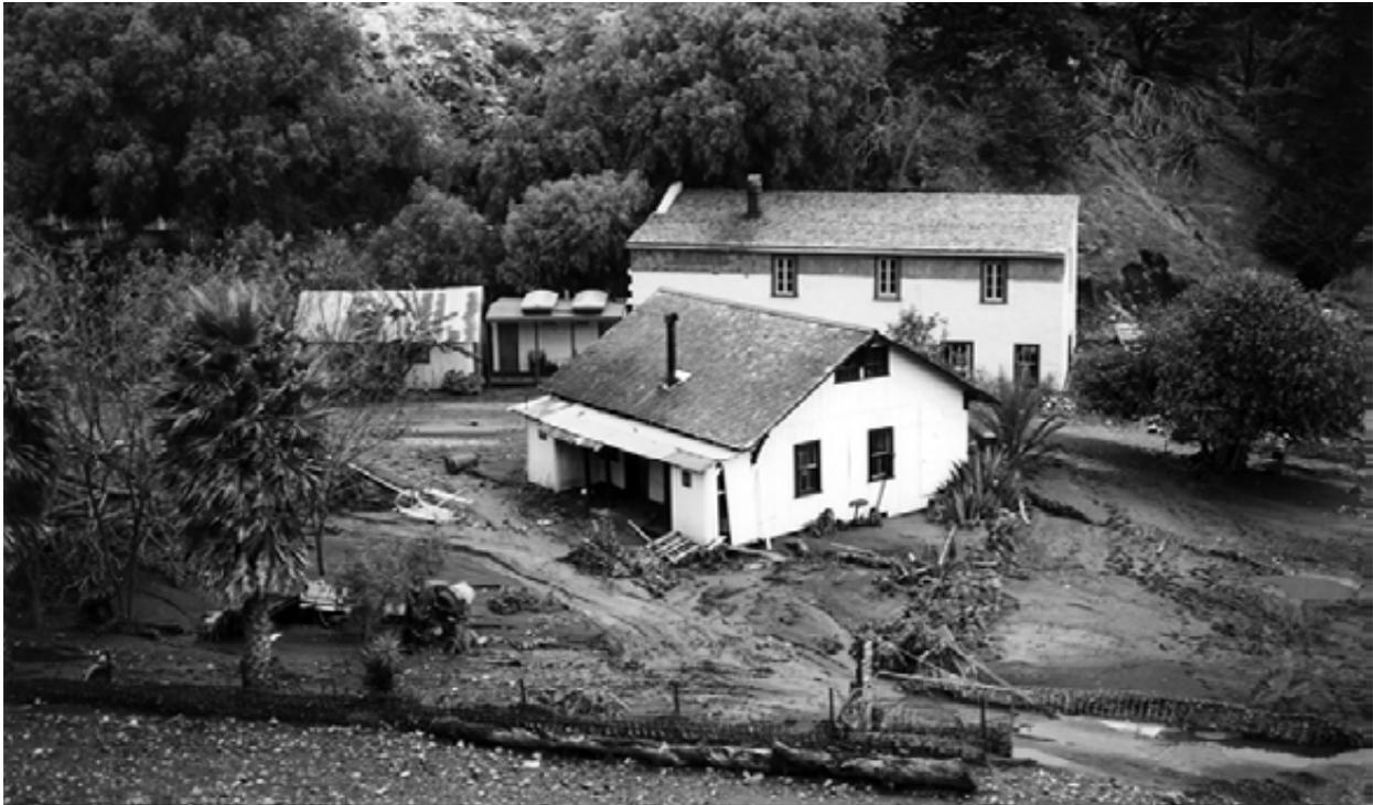
Figure 8-5. Scorpion Ranch after the flood of December 5–6, 1997. The intense flow twisted the bunkhouse off its foundation and wiped out the blacksmith shop.
