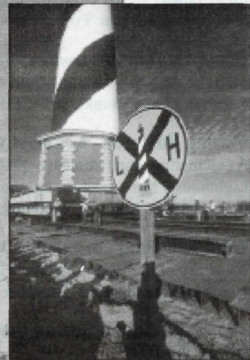
Traffic stops while the lighthouse crosses the four-way intersection.
