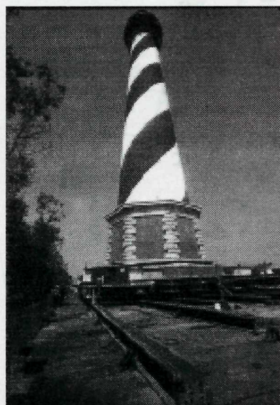
The Cape Hatteras Lighthouse and its move platform glide over the travel beams to the new home 1,600 feet from the ocean's edge.
