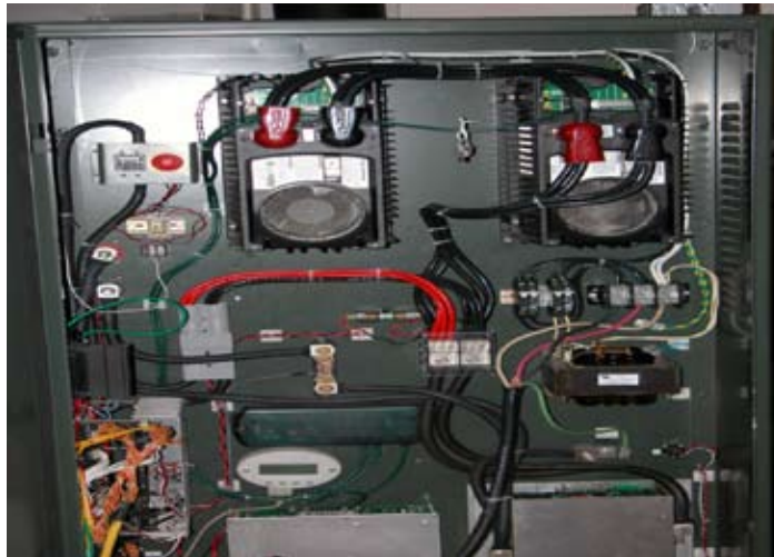
Kenai Fjords National Park tested a prototype propane fuel cell at Exit Glacier. NPS Photo
