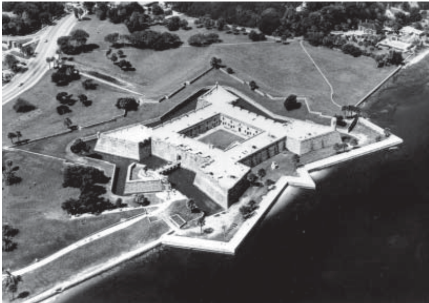
Aerial view of Castillo de San Marcos in St. Augustine Florida. Built by Spain from 1672 to 1695 the present fort is constructed of blocks of coquina and replaced nine successive wooden forts which had protected the city since its founding in 1565. Photo courtesy of Castillo de San Marcos National Monument.
