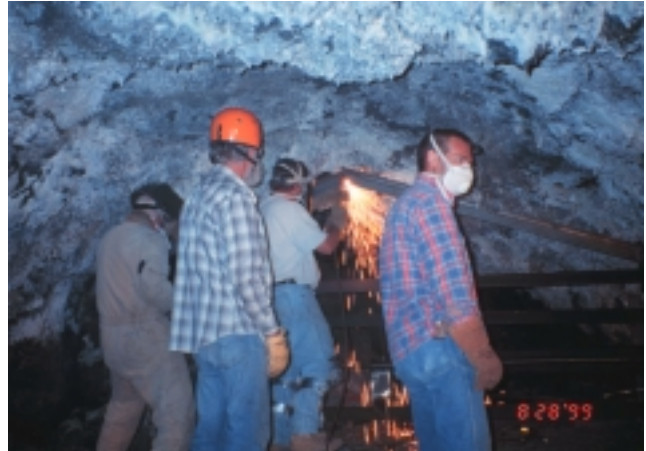
Welding on the gate in Arco Tunnel . (NPS Photo)
