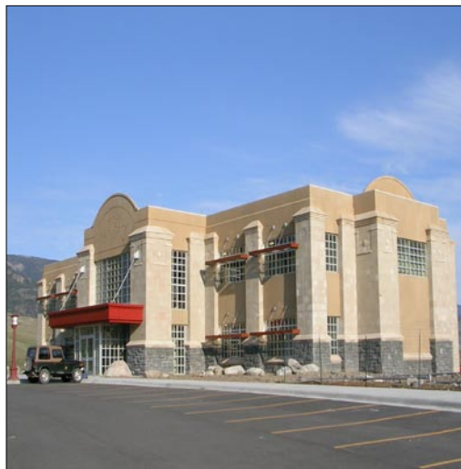
The awning-like structures of the Yellowstone Heritage and Research Center direct sunlight into the building's corridors where heat is stored in heat wells. Heating and cooling costs are correspondingly lower in this structure built with sustainability in mind.
