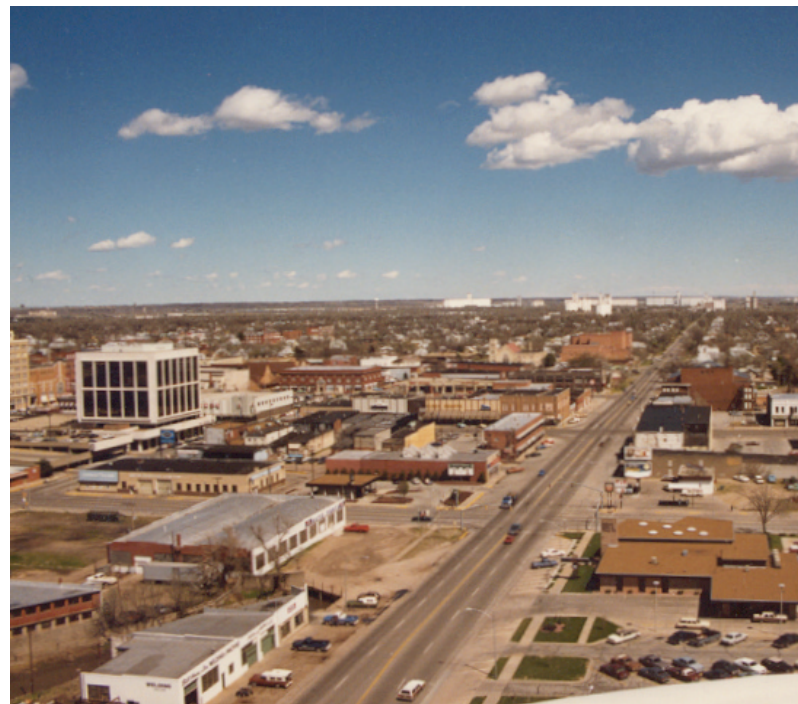
Avenue A in Hutchinson, Kansas before daylighting Cow Creek. This area frequently flooded during winter storms.
