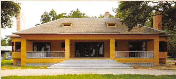
Exterior of the newly restored house
