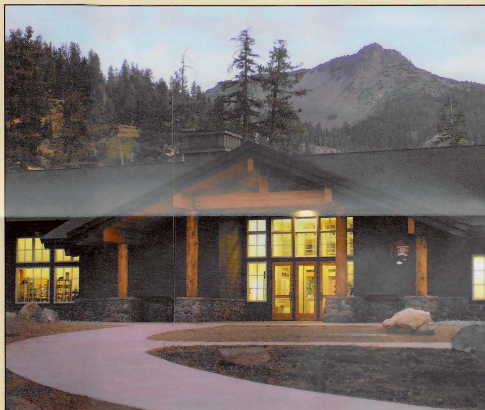
The new Lassen Volcanic National Park Kohm Yah-mah-nee Visitor Center received LEED Platinum certification, the highest level obtainable under the US Green Building Council's rating system. Other parks that are using LEED criteria in building designs include the USS Arizona Memorial, Redwood National and State Parks, Lake Mead National Recreation Area, and Mount Rainier National Park.
